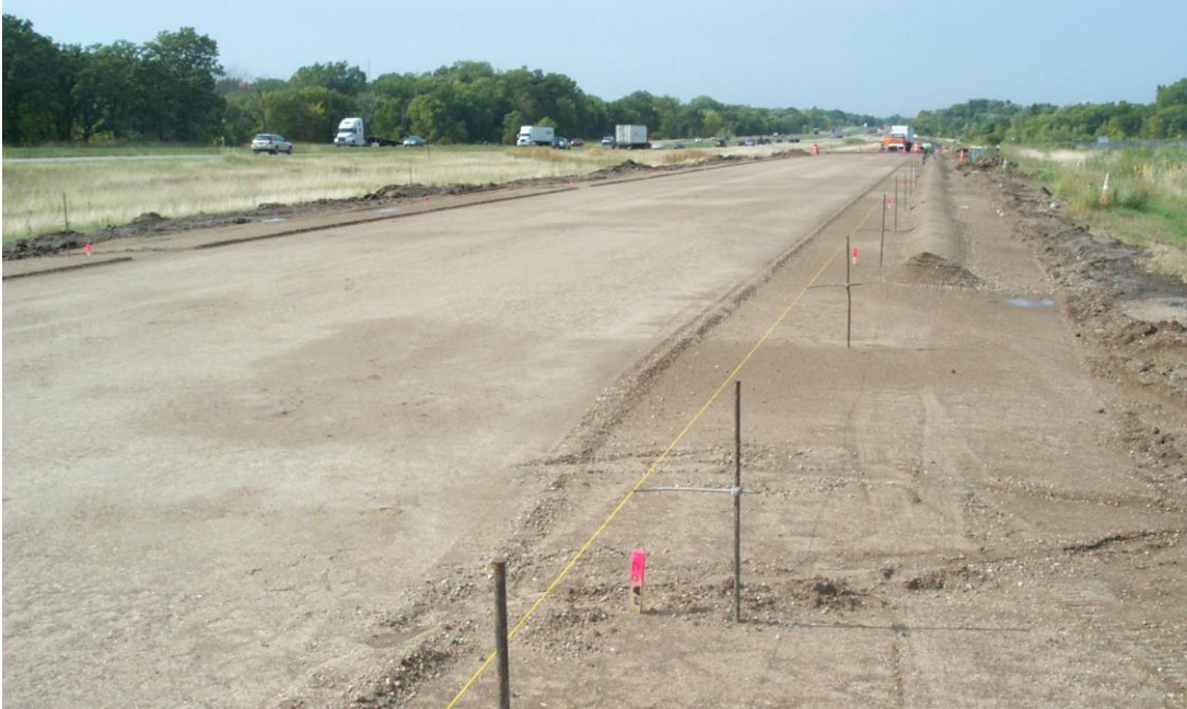
Figure 3.4 : Stringlines at 25 ft Interval. This is Typical
