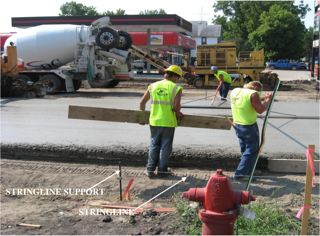
Figure 3.5: Stringlines In Close-Up
