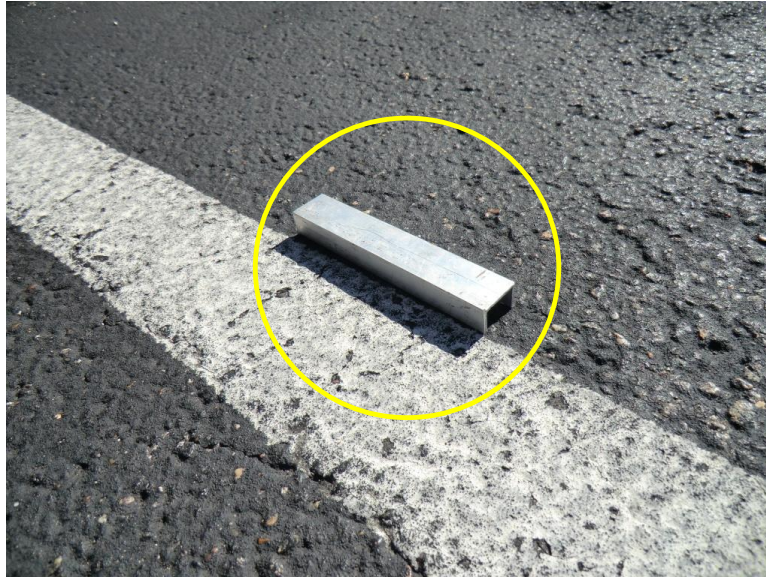
Figure 2-3. Aluminum channel used to mark the test section boundaries.
