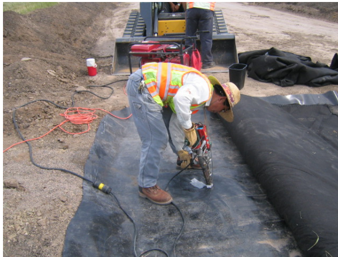
Figure 2. Installation of Lysimeter
