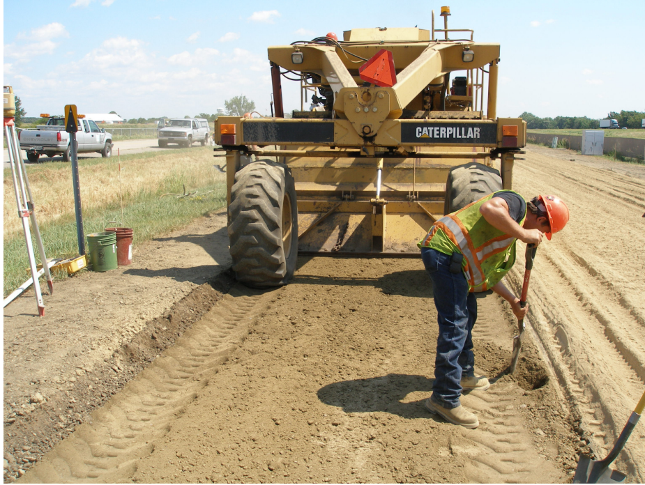
Figure 3. Placement and Mixing of Fly Ash
