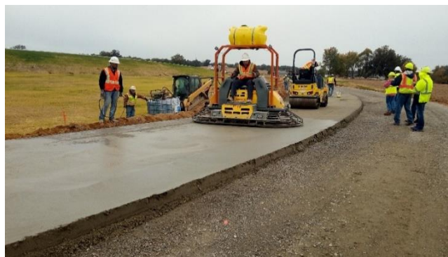
Figure 12 - Finishing process
