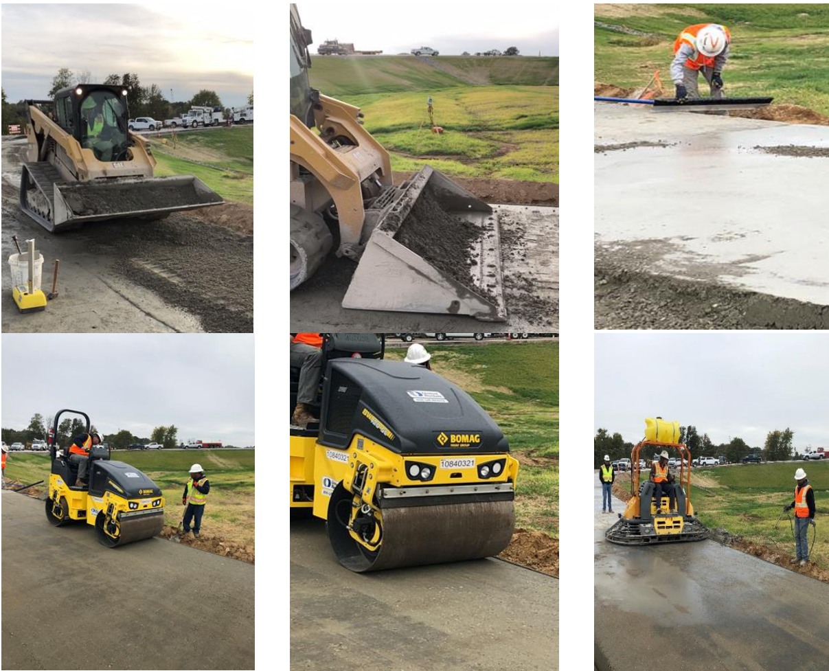
Figure 5 - Density adjustments
