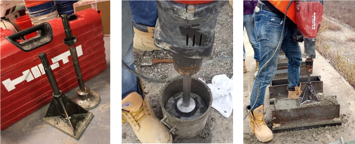
Figure 16 - Compaction tools and process
