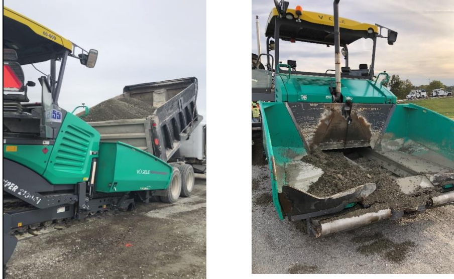
Figure 10 - Loading process of the slip-form paving
