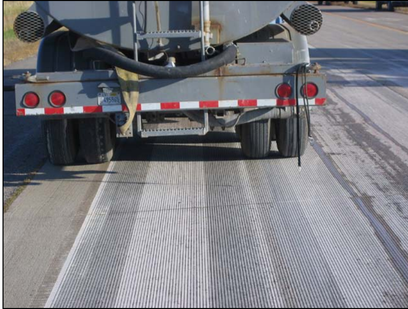
Figure 4.10. Ultimate grind (Cell 9) immediately behind the grinding machine.
