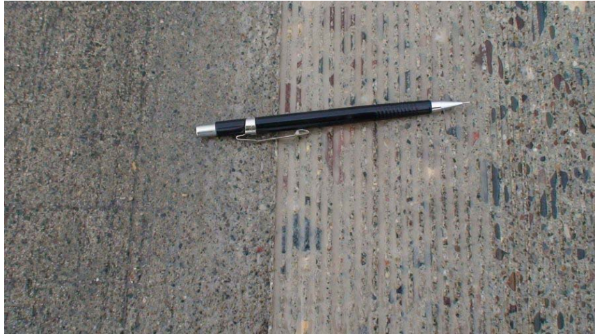
Figure 4.3. Conventional grind configuration (0.125X 0.125x0.120).
