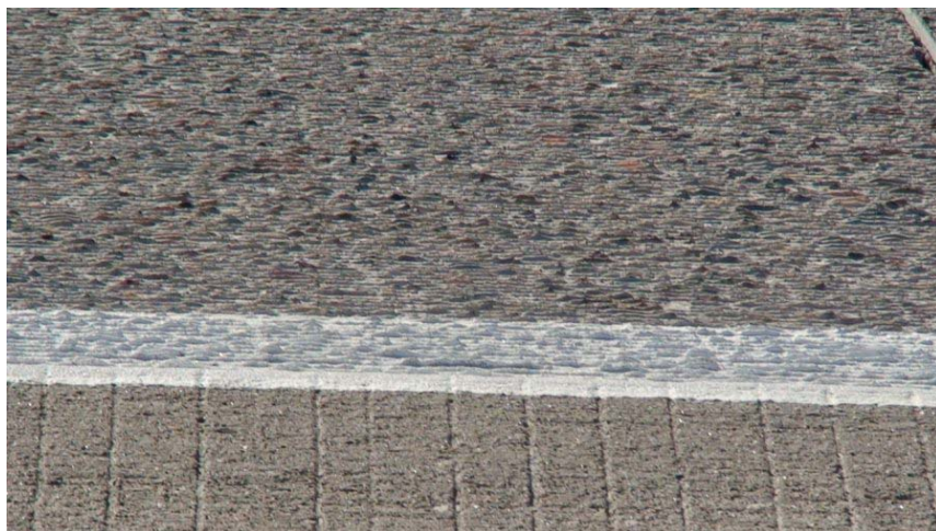
Figure 4.5. Conventional grind on Cell 8 and original transverse tining.
