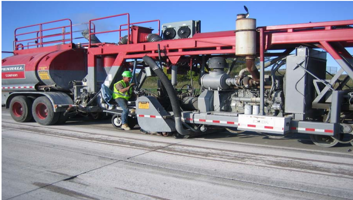
Figure 4.9. The ultimate diamond grinding process.
