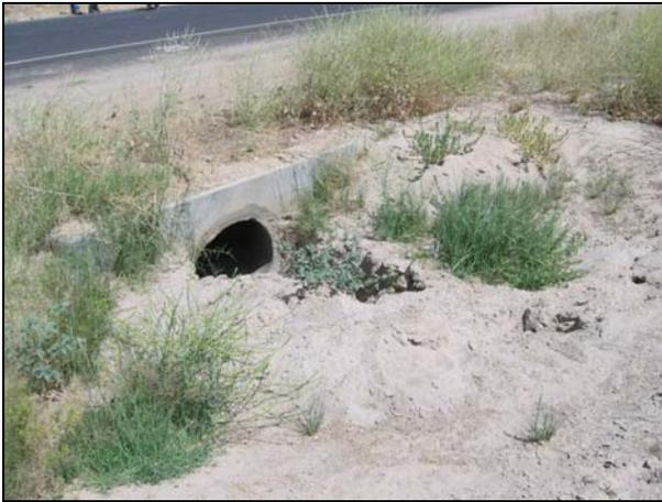
**Figure 4.19: Blocked culvert on 05-SB,SLO-33.**
