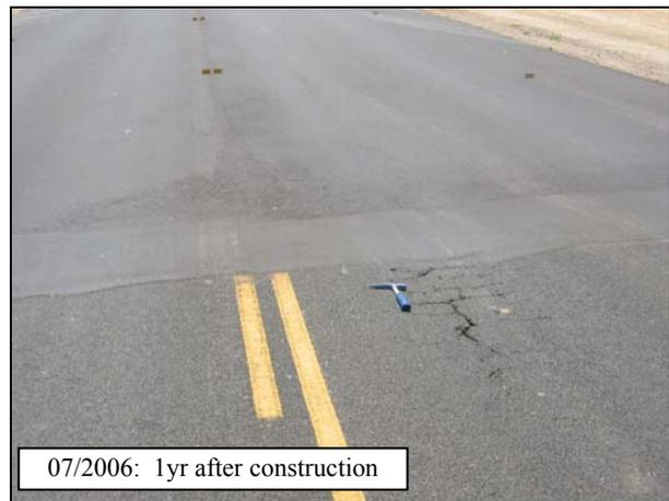
**Figure 4.17: New distress next to digout on 05-SB,SLO-33 (July 2006).**
