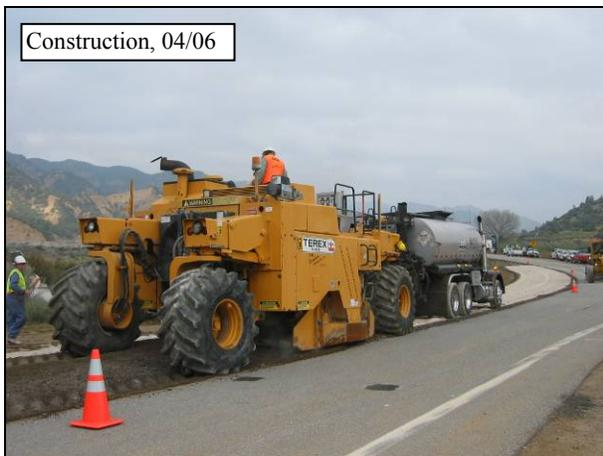
**Figure 4.45: Foamed asphalt injection (Train 1) on 07-VEN-33.**
