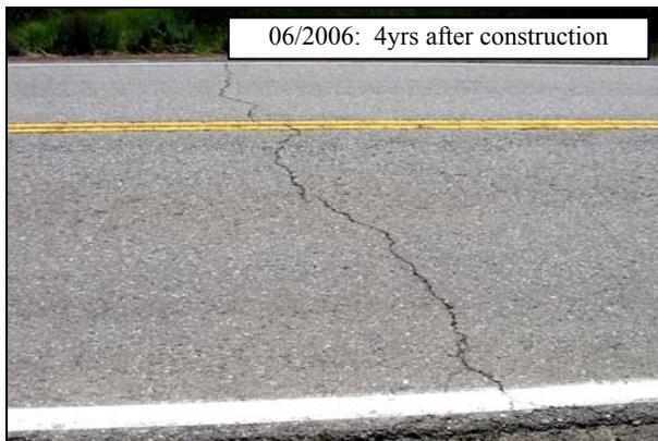
**Figure 4.9: Thermal cracking on 03-SIE-89.**
