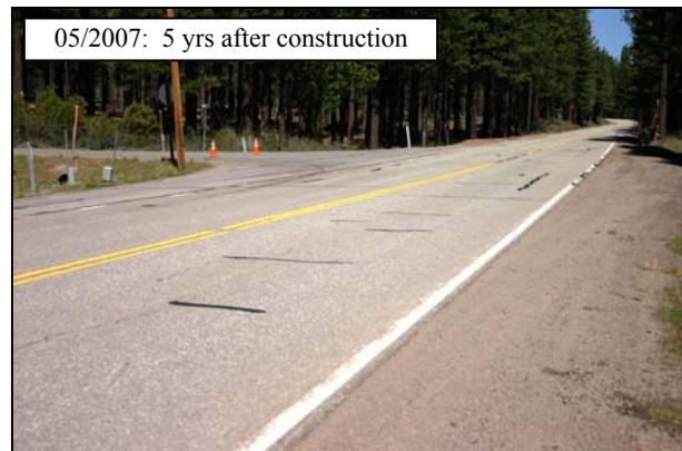
**Figure 4.10: Sealed transverse cracks on 03-SIE-89.**
