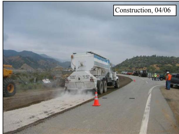
**Figure 4.44: Cement kiln dust application on 07-VEN-33.**
