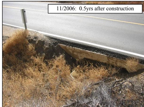
**Figure 4.64: Blocked drain. (1) on 07-VEN-33.**
