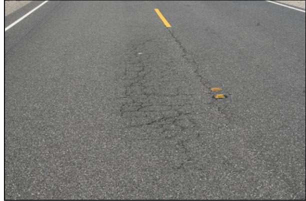
**Figure 4.3: Fatigue Cracking in inner wheelpath on 03-COL-20 (2007).**
