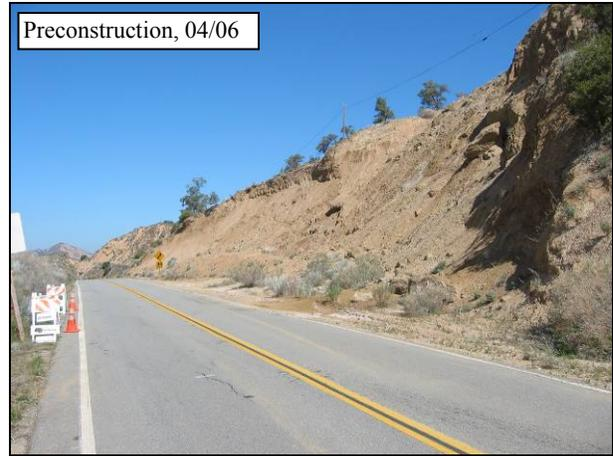
**Figure 4.37: Preconstruction cracking associated with slope instability on 07-VEN-33.**
