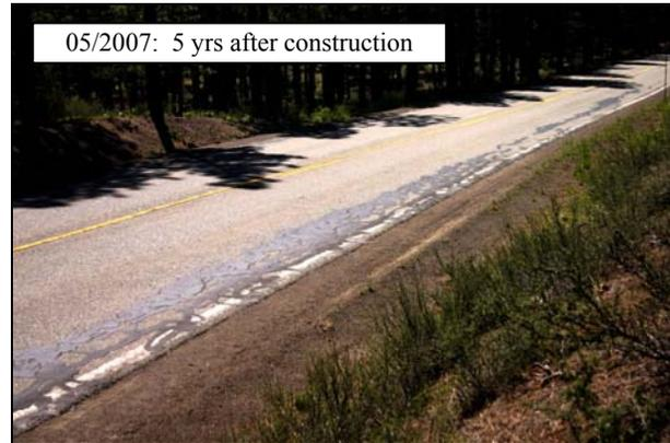
**Figure 4.8: Sealed outer wheelpath cracks on 03-SIE-89.**
