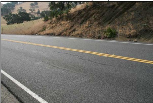
**Figure 4.6: Longitudinal cracks in hill section on 03-COL-20 (2007–2008).**
