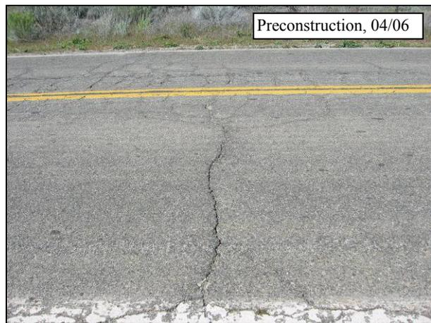
**Figure 4.35: Preconstruction transverse cracking on 07-VEN-33.**
