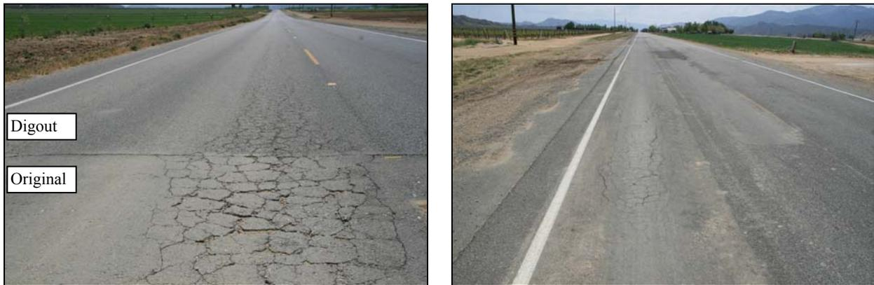
**Figure 4.27: New distress on previous digout on 05-SB,SLO-33 (May 2008).**
