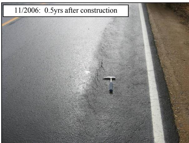
**Figure 4.59: Shearing in the asphalt concrete on 07-VEN-33.**
