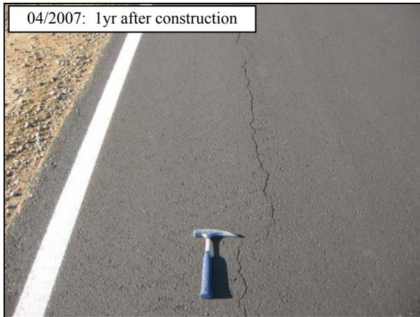
**Figure 4.66: Longitudinal cracking on 07-VEN-33 (April 2007).**
