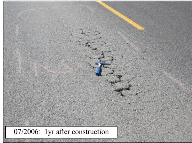
**Figure 4.15: Severe distress (3) on 05-SB,SLO-33 (July 2006).**
