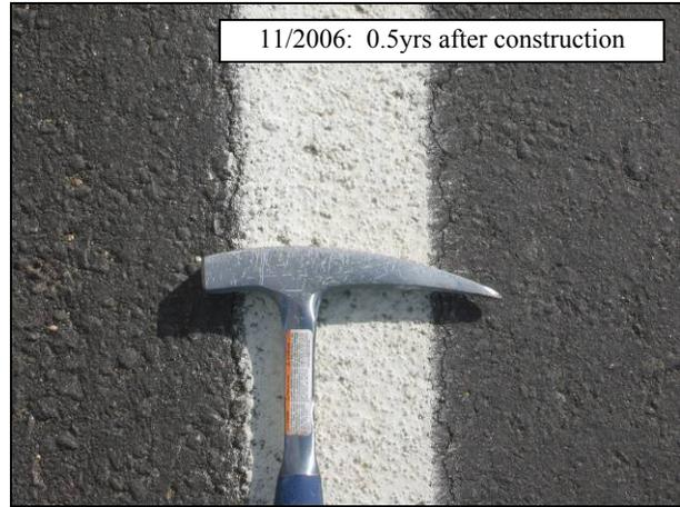
**Figure 4.62: Cracking around edge striping on 07-VEN-33.**
