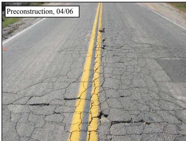
**Figure 4.34: Preconstruction fatigue (alligator) cracking on 07-VEN-33.**
