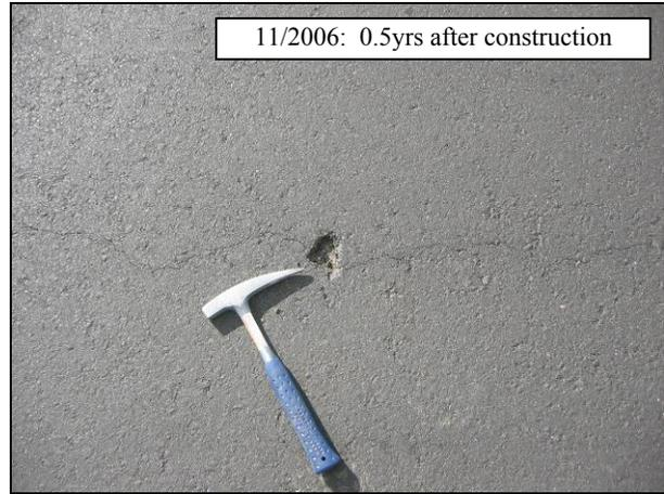
**Figure 4.57: Longitudinal crack and loss of oversize stone on 07-VEN-33.**
