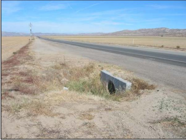
**Figure 4.18: Filled in side drains on 05-SB,SLO-33.**
