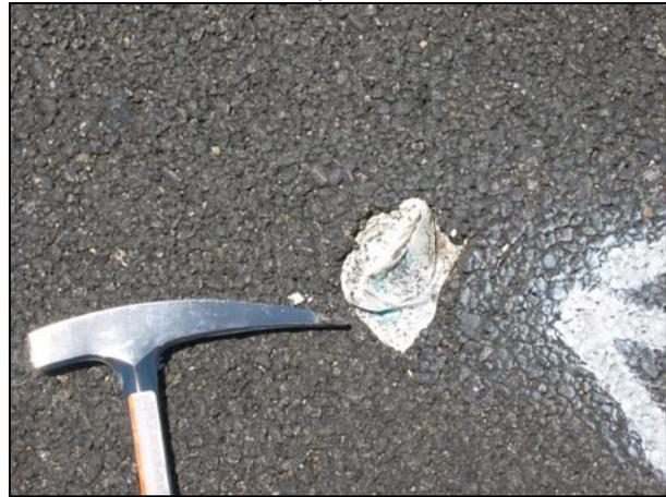
**Figure 4.25: Trash compacted into asphalt concrete on 05-SB,SLO-33.**
