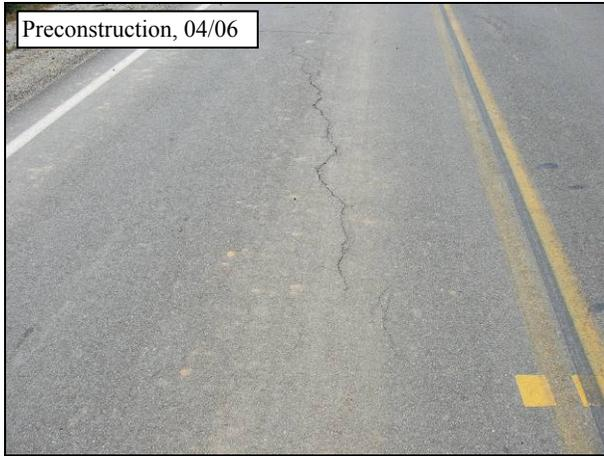
**Figure 4.36: Preconstruction longitudinal cracking on 07-VEN-33.**
