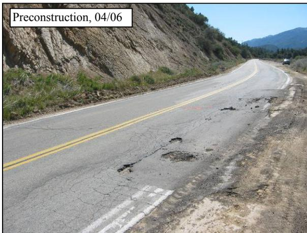
**Figure 4.38: Preconstruction patching on 07-VEN-33.**
