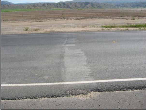
**Figure 4.22: Poor construction joint on 05-SB,SLO-33.**
