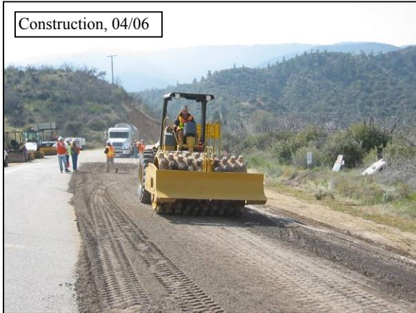
**Figure 4.47: Initial compaction with padfoot roller on 07-VEN-33.**
