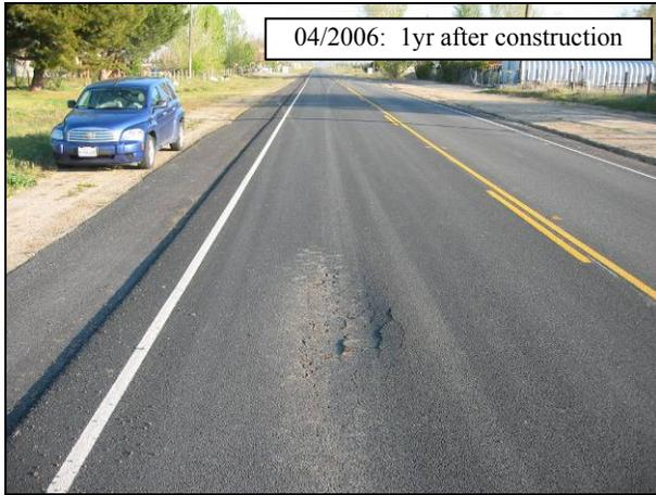
**Figure 4.14: Severe distress (2) on 05-SB,SLO-33 (April 2006).**
