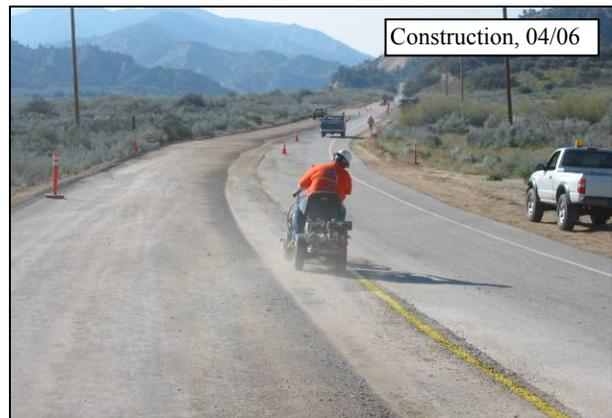
**Figure 4.52: Temporary striping application on 07-VEN-33.**
