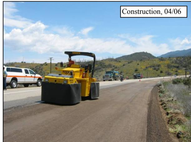
**Figure 4.50: Final compaction with rubber-tired roller on 07-VEN-33.**
