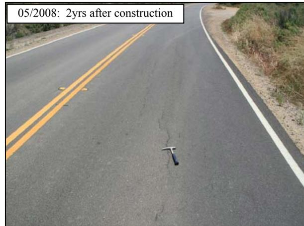
**Figure 4.67: Longitudinal cracking on 07-VEN-33 (May 2008).**
