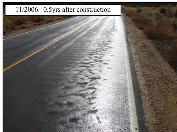
**Figure 4.60: Roughness in asphalt concrete on 07-VEN-33.**
