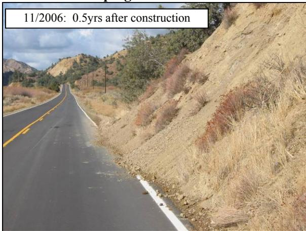
**Figure 4.63: Debris from slope instability on 07-VEN-33.**
