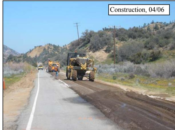
**Figure 4.48: Water application behind recycling train on 07-VEN-33.**
