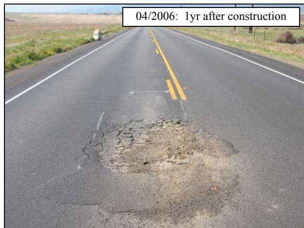
**Figure 4.13: Severe distress (1) on 05-SB,SLO-33 (April 2006).**
