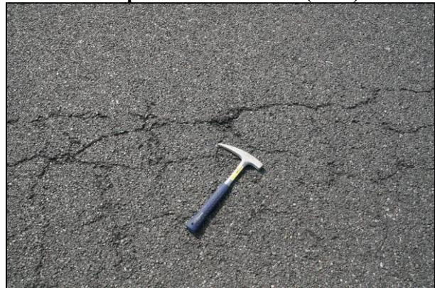
**Figure 4.5: Spalled cracks through open-graded friction course on 03-COL-20 (2008).**
