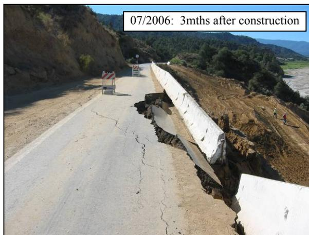
**Figure 4.68: Damage associated with landslide (July 2006).**
