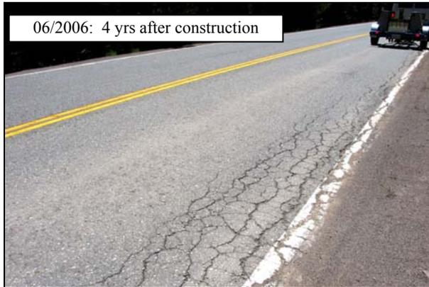
**Figure 4.7: Outer wheelpath cracking on 03-SIE-89.**
