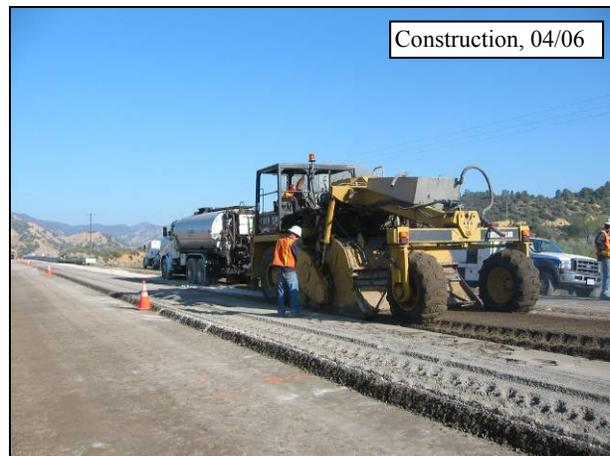
**Figure 4.46: Foamed asphalt injection (Train 2) on 07-VEN-33.**
