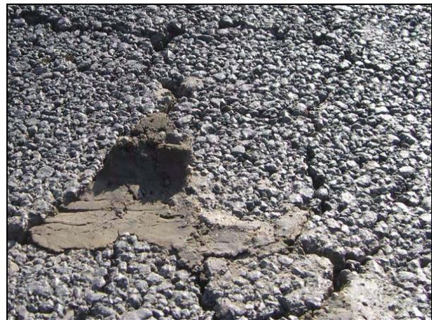
Figure 4.33: Fines pumped through base and asphalt concrete.
