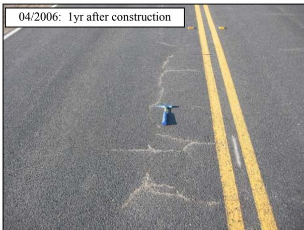
**Figure 4.12: Early cracking with pumping on 05-SB,SLO-33 (April 2006).**
