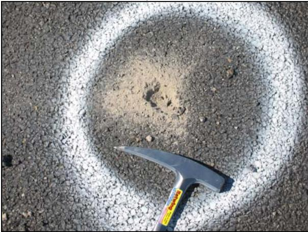
**Figure 4.24: Area of thin asphalt concrete on 05-SB,SLO-33.**
