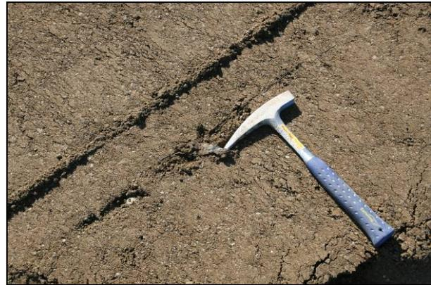
**Figure 7.31: Asphalt strings in recycled material.**
