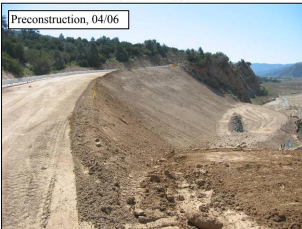
**Figure 4.40: Pre-construction landslide repair on 07-VEN-33.**
