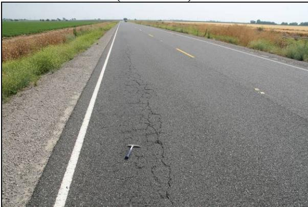
**Figure 4.4: Fatigue cracking in outer wheelpath on 03-COL-20 (2008).**
