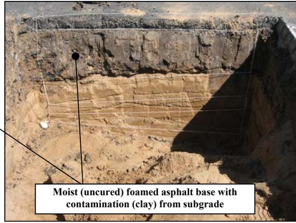
Figure 4.30: Test pit #2 on 05-SB,SLO-33.
