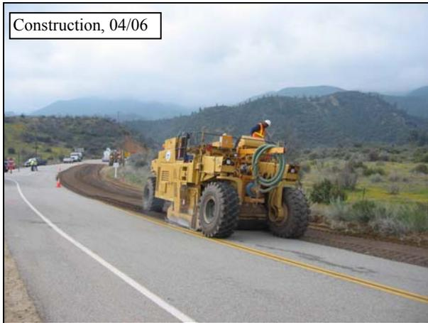
**Figure 4.43: Prepulverization on on 07-VEN-33.**
