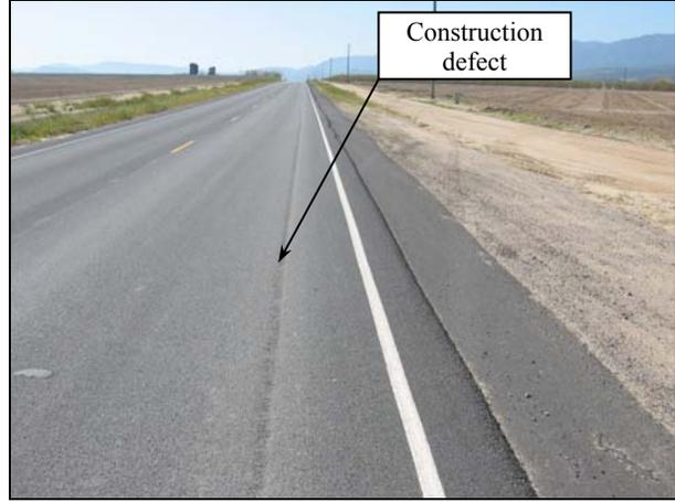
**Figure 4.23: Construction defect on 05-SB,SLO-33.**
