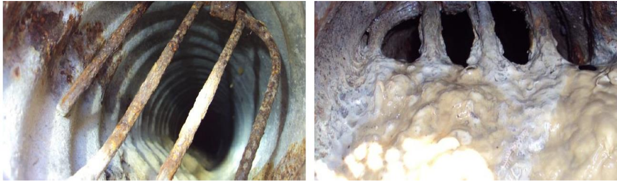
Figure 4.1. Clean pipe (left) and partially clogged pipe (right) (Ceylan et al. 2013)
