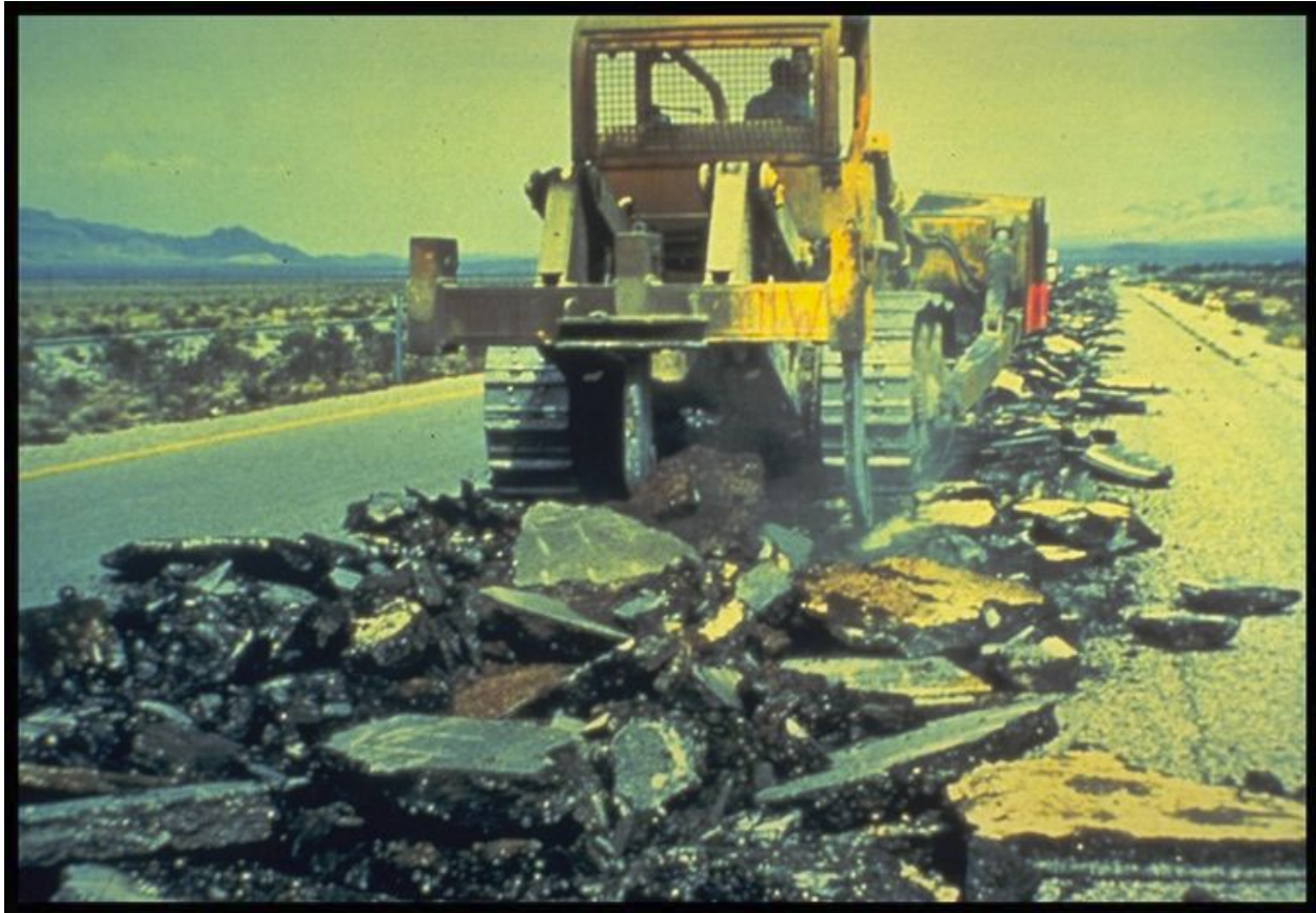
Figure 1.1 Dozer with ripper-tooth (Kandhal and Mallick, 1997).
