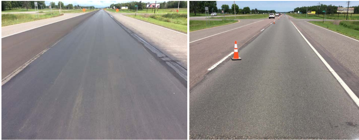
Cell 169022: As constructed in 2016 (left) and inspected 7-16-19 (right).
