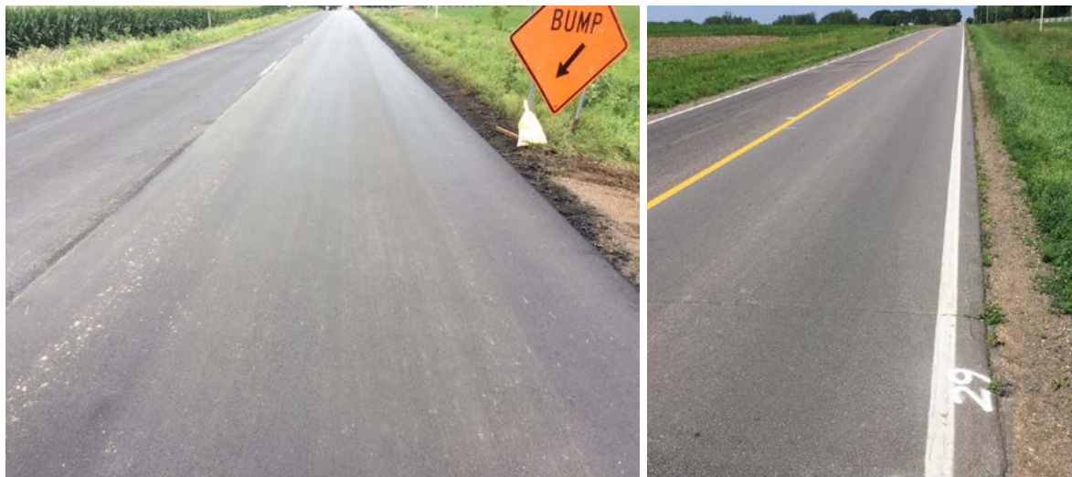
Cell 8029: As constructed in 2016 (left) and inspected 7-15-19 (right).
