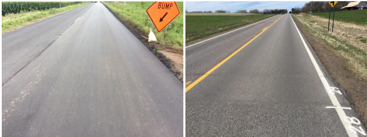
Cell 8029 Thinlay with Delta-S: As constructed in 2016 (left) and inspected 4-28-21 (right).
