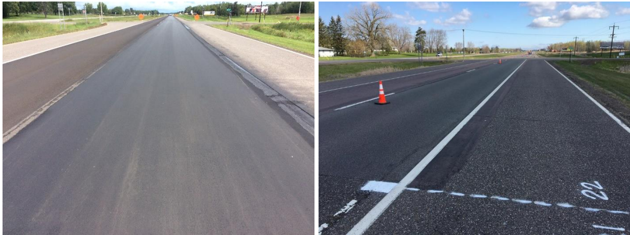
Cell 169022 Thinlay with Delta-S: As constructed in 2016 (left) and inspected 4-29-21 (right).
