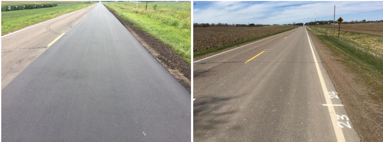
Cell 8024 Thinlay No Delta-S as constructed in 2016 (left) and inspected 4/28/21 (right).
