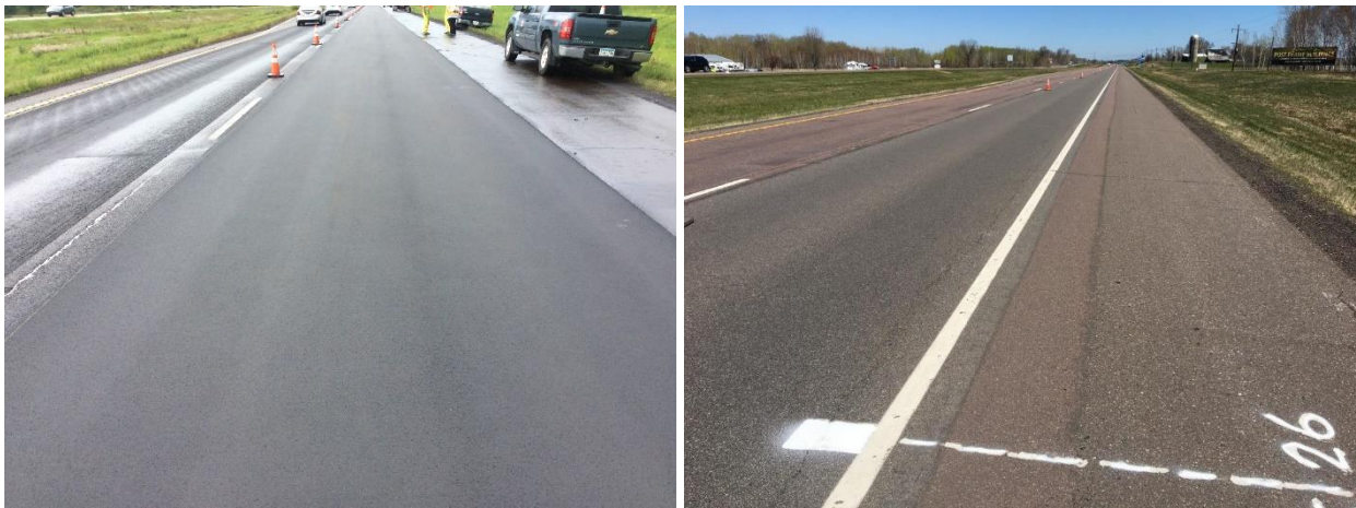
Cell 169026 Thinlay No Delta-S as constructed in 2016 and inspected 4-29-21 (right).
