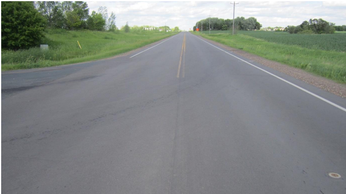
Figure 10 View eastbound into sections 7006E and 7006W, June 2020.
