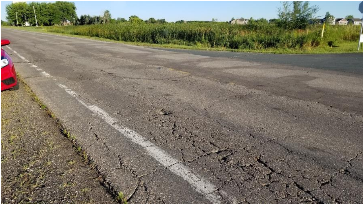
Figure 1 70th St. August 2019. Eastbound (left), and westbound (right) lanes.
