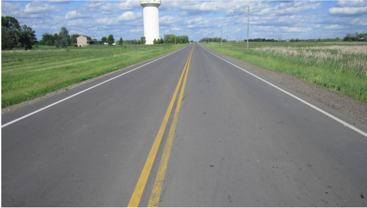
Figure 9 View eastbound into sections 7001E and 7001W, June 2020.
