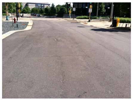
Figure 100.14 – Bituminous patch over raveled pavement.
