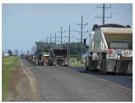
**Figure 600.36** – Excessively long truck queue. The bituminous mixture in the trucks waiting at the far end of the queue will likely have cooled to an unacceptable temperature by the time it gets to the paver.
