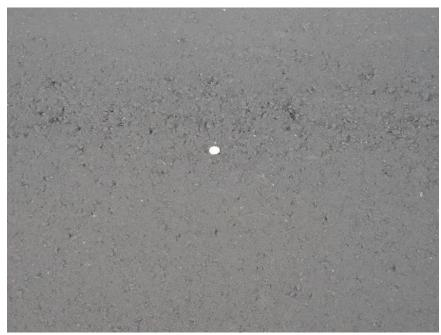
Figure 600.8 – Slightly segregated pavement
