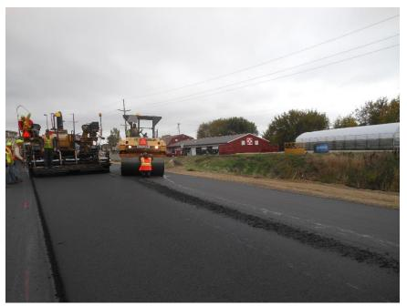
Figure 600.26 – Steel drum roller picking up mix.
