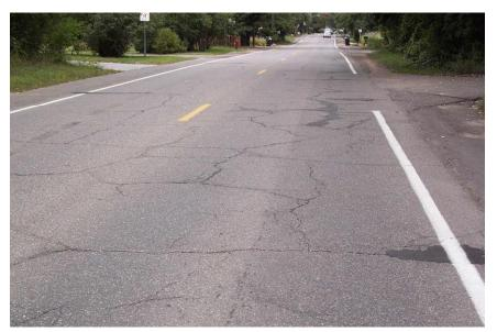
Figure 100.16 – Block Cracking
