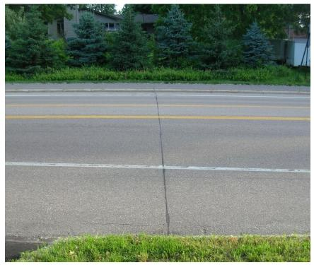
Figure 200.19 - Saw and Seal roadway
