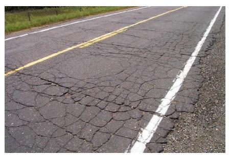
Figure 100.17 – Severe Fatigue Cracking
