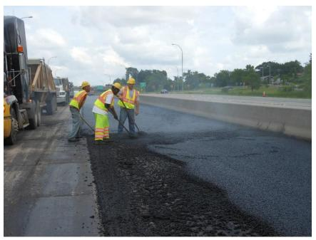
**Figure 600.21** – The result of "paving" without bituminous mixture present in the paver hopper
