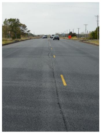
Figure 600.30 – Wavy Longitudinal Joint
