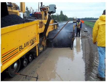
**Figure 600.34** – Paving in the rain. When the paver creates a wake through the water, it is well past time to halt production. The situation pictured above should never be allowed to occur.
