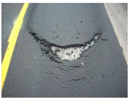
**Figure 600.40** – Longitudinal shoving of the bituminous mat as a result of insufficient or nonexistent tack coat. In this case, the wrong bituminous mixture was used for the application in addition to insufficient tack coat prior to paving.
