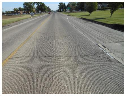
**Figure 500.2** – Chevron pattern after milling. Note the angled grooves in the milled surface.
