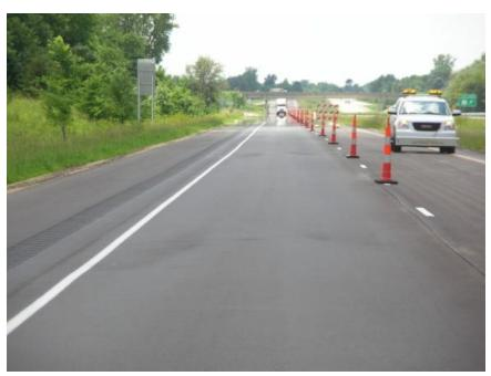
Figure 600.7 – Chevrons from folding hopper wings
