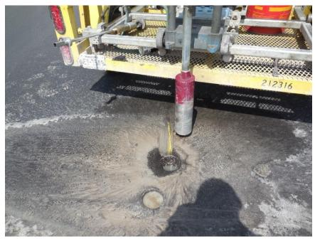
Figure 500.26 - Core Drill
