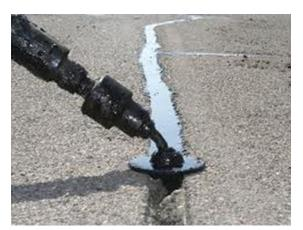
Figure 100.11 – Crack sealant applied from the wand.
