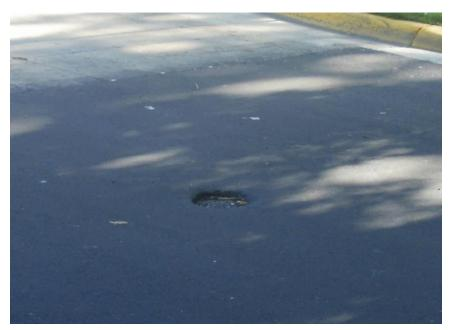
Figure 500.30 – Water valve box that has been adjusted too low.
