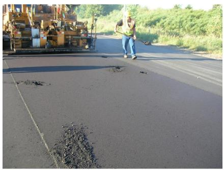
**Figure 600.38** – Removal of chunks from the bituminous mat. The areas will have to be filled in by hand, and will likely be areas of localized segregation. Paving operations should halt if this continues.
