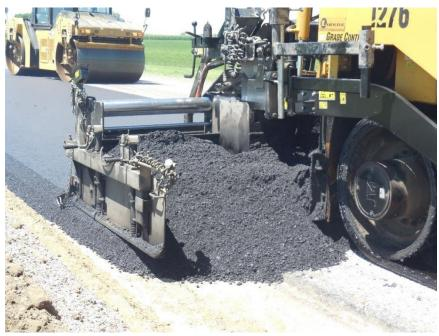
**Figure 600.18** – Excessive material head in front of the screed. The augers should not be buried.
