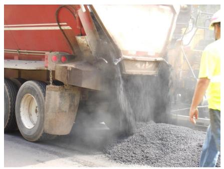
Figure 500.9 – A flow-boy windrows bituminous mix
