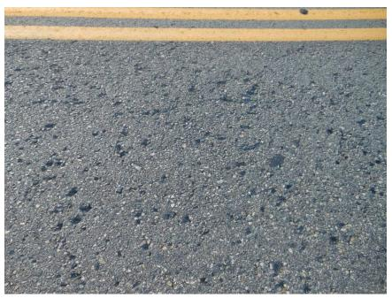
**Figure 600.17** – The result of excessive spall material in a mix. This may have a profound effect on the long-term durability of the pavement.
