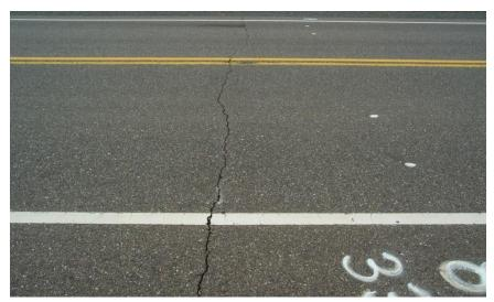
Figure 100.15 – Transverse Thermal Crack
