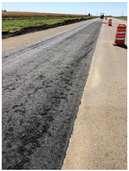
Figure 600.25 – Pneumatic Tired Roller picking up mix.
