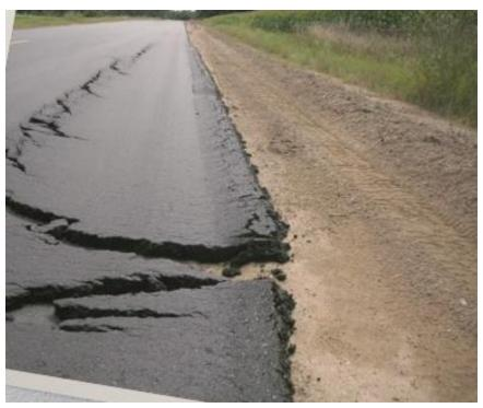
Figure 600.23 – Yielding of the aggregate base
