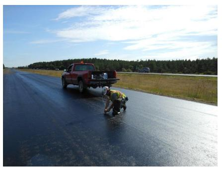
Figure 600.31 – Contractor setting stringline to guide the paver
