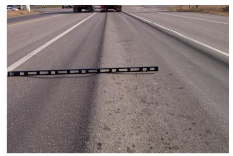
Figure 100.18 - Pavement Rutting
