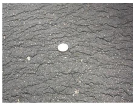
Figure 600.22 - Checking of the mat
