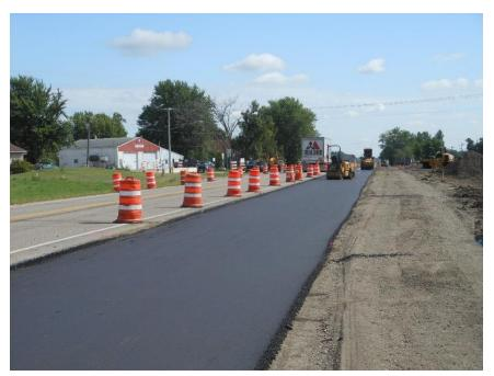
Figure 500.1 – Paving operation within a traffic control setup.
