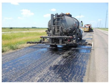
**Figure 500.6** – Tack coat distributor truck. Note the streaked appearance. The Contractor should respray this area to achieve uniform coverage.
