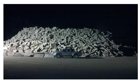
Figure 200.14 – Pile of recycled concrete ready for crushing
