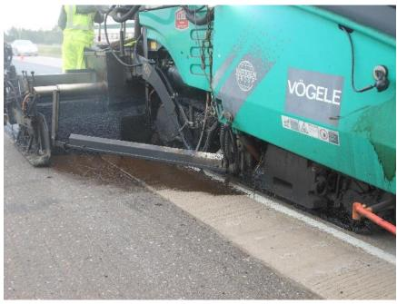
Figure 100.2 – Spray paver applying tack and UTBWC
