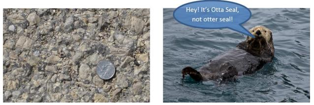
Figure 100.9 – Bituminous Otta Seal (Left). Not a Bituminous Otta Seal (Right). Otter image credit: NPS/K. Thoresen
