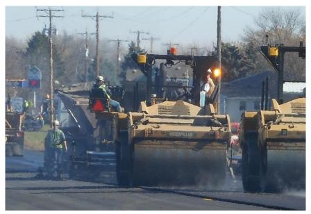
**Figure 500.22** – Compacting an unconfined edge. Note the roller at the front of the train hanging the drum over the edge by several inches.
