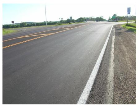
Figure 100.8 – Micro Surfacing
