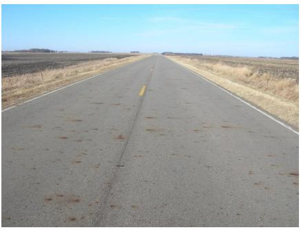
Figure 600.16 – The effect of excessive Iron Oxide in the bituminous mixture.
