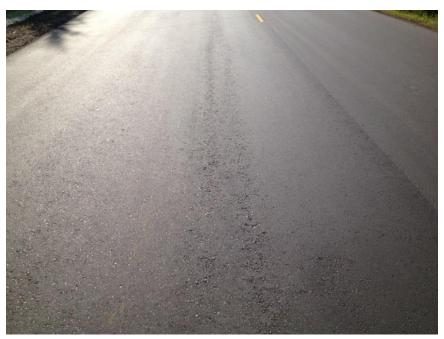
Figure 600.9 – Moderate segregation of the pavement
