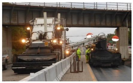
**Figure 500.13** – A Material Transfer Vehicle delivers bituminous mixture to the paver. Note that, due to space limitations around the paver, the MTV is in an adjacent lane to the paver. This allows the haul trucks more room to deliver the mix to the MTV.
