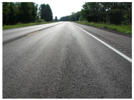
Figure 600.10 – Severely segregated pavement
