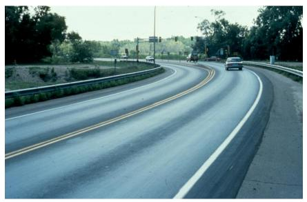
Figure 600.11 – Pavement Flushing
