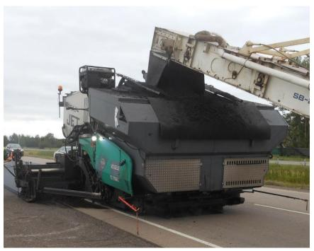
**Figure 500.17** – Spray paver in action. Note the tack coat spray bars in front of the screed.
