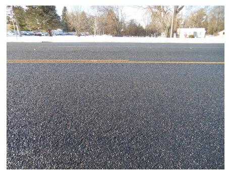
Figure 100.7 – Bituminous Seal Coat
