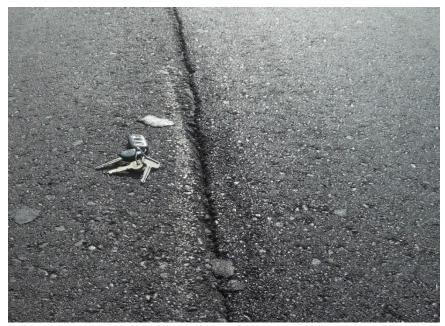
Figure 600.32 – Poorly compacted longitudinal joint
