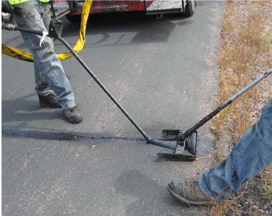
Figure 7 – Typical filling of squeegee for leveling operations (1ft. squeegee pictured)
