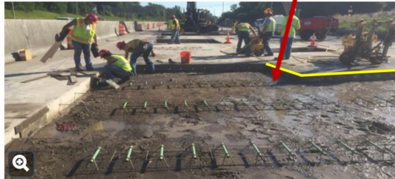
Type CD-HV +Type CX Repair Installation of Dowel Bar Baskets
