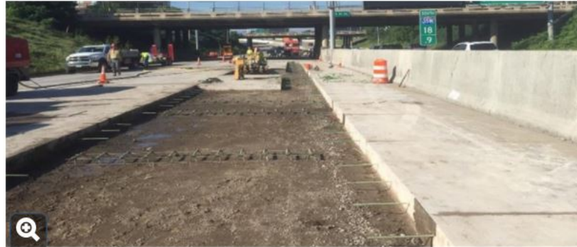
Type CD-HV +Type CX Repair Installation of Dowel Bar Baskets
