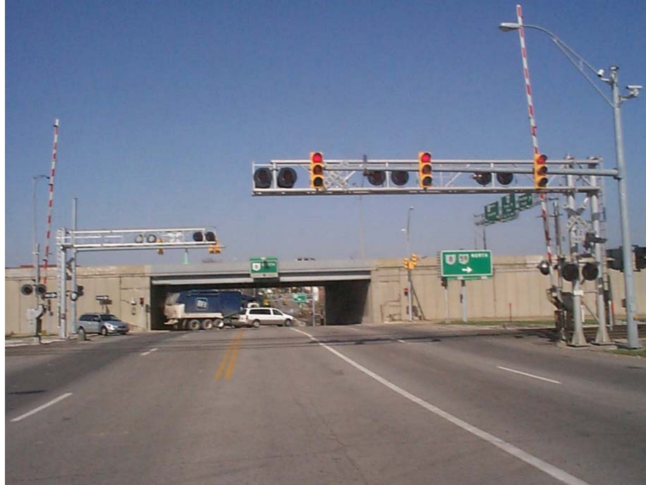
Figure 4 Grade Crossing with Traffic Signal Preemption (Source: Public Utilities Commission of Ohio Grade Crossing Inventory, http://www.ohiorail.ohio.gov/crossings.php )
