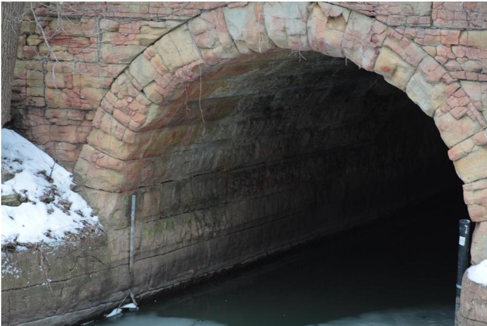
View facing south-southwest, showing close-up of tunnel outlet and stone masonry arch
