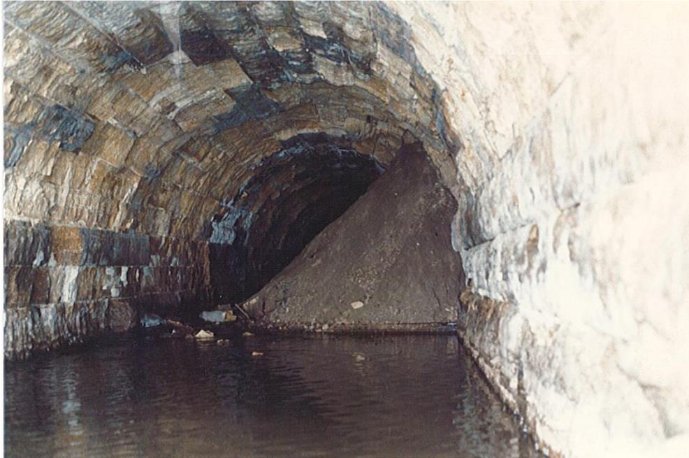
View facing southwest; 1989 photograph showing stone masonry and partial washout
