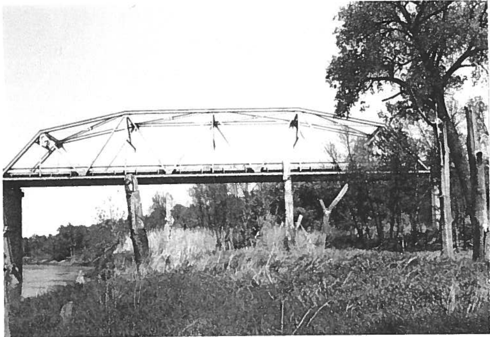
Elevation of eastern truss, facing north.
