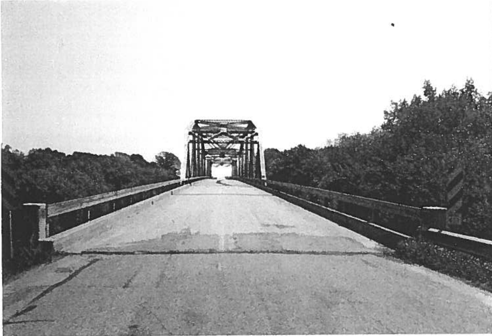
Portal view, facing east.
