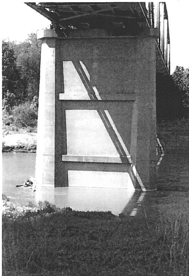
Center pier, facing west-southwest.
