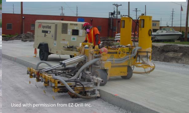
BMP 6. Dust vacuum system attachment to 4 gang dowel drill machine in full operation.
