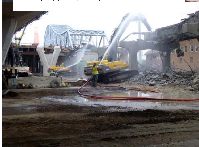
BMP 7. Comparison between water mister on jack hammer operation to high pressure/volume canon spray (TH35, TH61).
