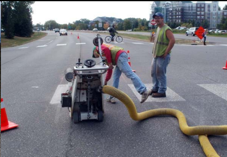
BMP 3/4. Good examples of pavement marking grinding using appropriately sized vacuum systems, scaled to the work. Vacuum hoppers require high maintenance and care to prevent loss during handling.
