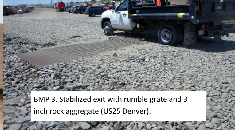
BMP 3. Stabilized exit with rumble grate and 3 inch rock aggregate (US25 Denver).
