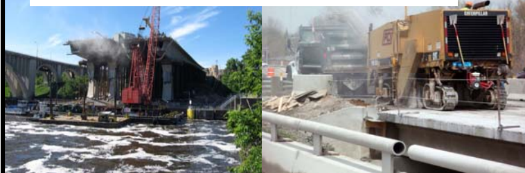
Dust controls on surface preparations require pre- and post planning for all related activities to ensure bonding compatibility.
