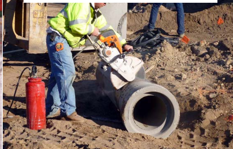
BMP 2. Apply appropriate water from pressure tank to saw fitting (University Ave Light Rail)
