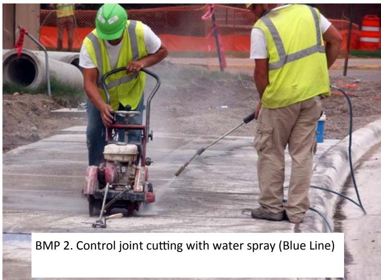
BMP 2. Apply appropriate water from pressure tank to saw fitting (University Ave Light Rail)
