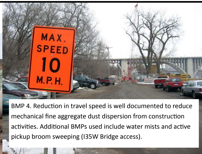
BMP 4. Reduction in travel speed is well documented to reduce mechanical fine aggregate dust dispersion from construction activities. Additional BMPs used include water mists and active pickup broom sweeping (I35W Bridge access).
