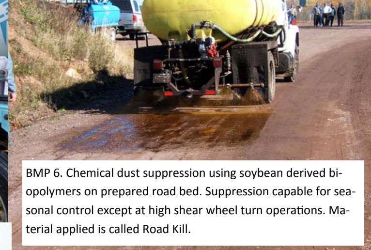
BMP 6. Chemical dust suppression using soybean derived bi-polymers on prepared road bed. Suppression capable for seasonal control except at high shear wheel turn operations. Material applied is called Road Kill.
