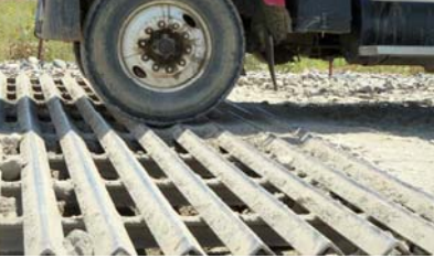
BMP 4. Exit Control Type Rumble Pad
