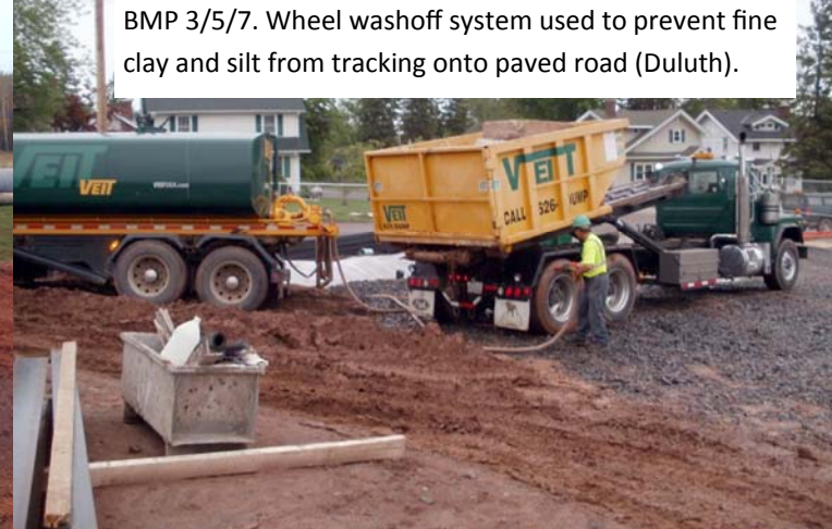
BMP 3/5/7. Wheel washoff system used to prevent fine clay and silt from tracking onto paved road (Duluth).
