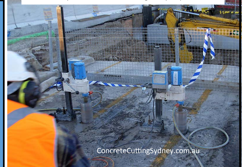
BMP 4/5. Wet drill hole (TH610 T1 rail) drilling and active vacuum slurry removal or core cutting slurry trap wall.
