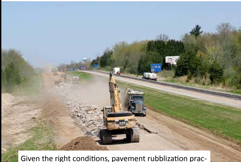
Given the right conditions, pavement rubblization practices are typically less dust prone than backhoe removal, truck loading, and hauling
