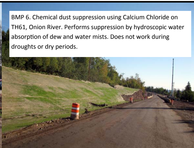
BMP 6. Chemical dust suppression using Calcium Chloride on TH61, Onion River. Performs suppression by hygroscopic water absorption of dew and water mists. Does not work during droughts or dry periods.
