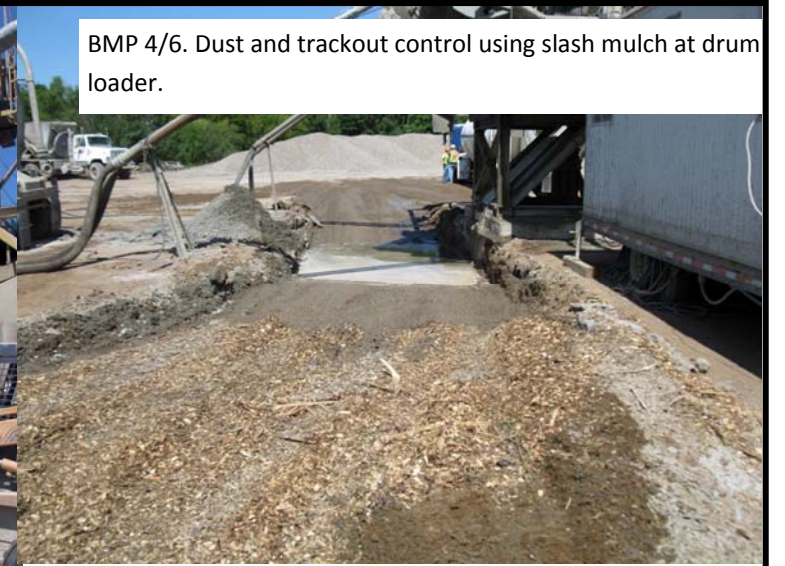
BMP 4. TH35 Harris Batch plant watering slash mulch exit using treated salvaged water. (TH35)
