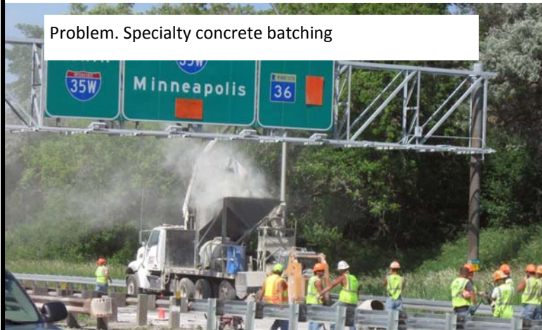
BMP 8. Install plastic wind shield over Portland cement loading hopper. (TH61 Overlook)
