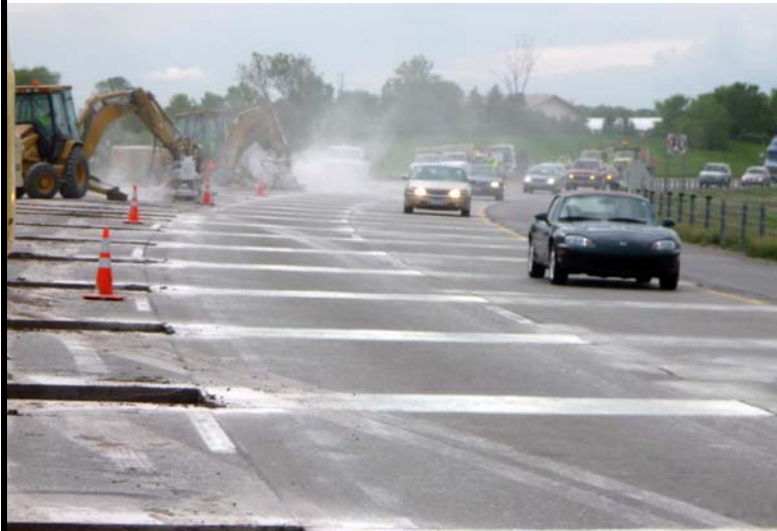
Problem. Dowel bar drilling for pavement rehabilitation
