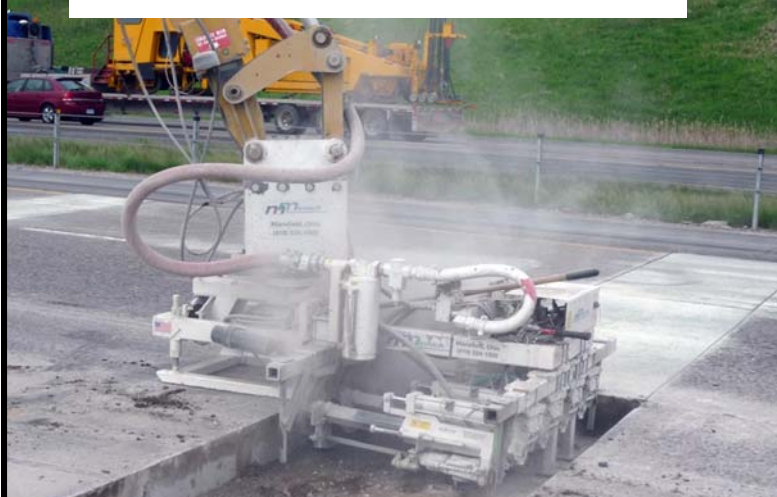
Problem. Dowel bar drilling for pavement rehabilitation
