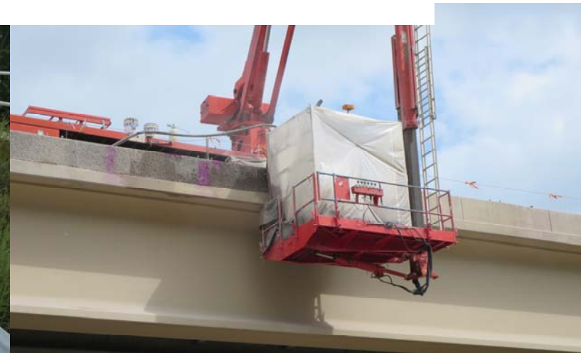
BMP 2/7. Material capture shroud containment over river.
