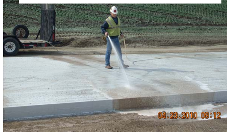
BMP 4. Wash pavement that removes material to shoulder area entrapment prior to becoming dust problem (TH35). Slurry material directed to future shoulder entombment.
