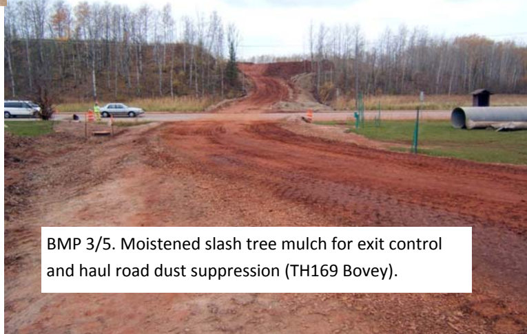
BMP 3/5. Moistened slash tree mulch for exit control and haul road dust suppression (TH169 Bovey).
