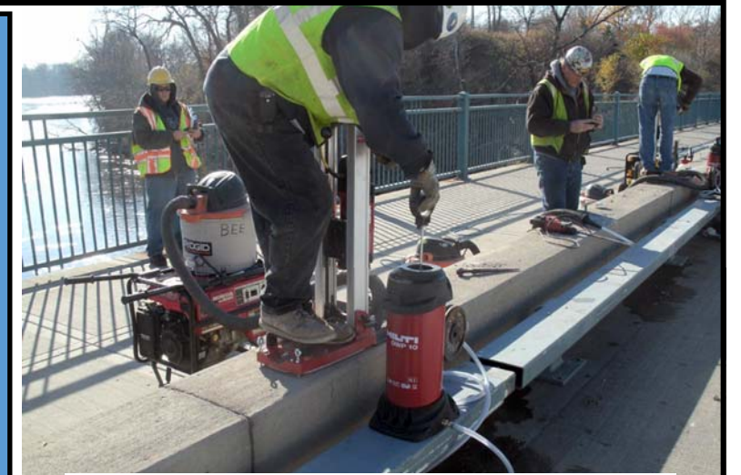
BMP 4/5. Wet drill hole (TH610 T1 rail) drilling and active vacuum slurry removal or core cutting slurry trap wall.
