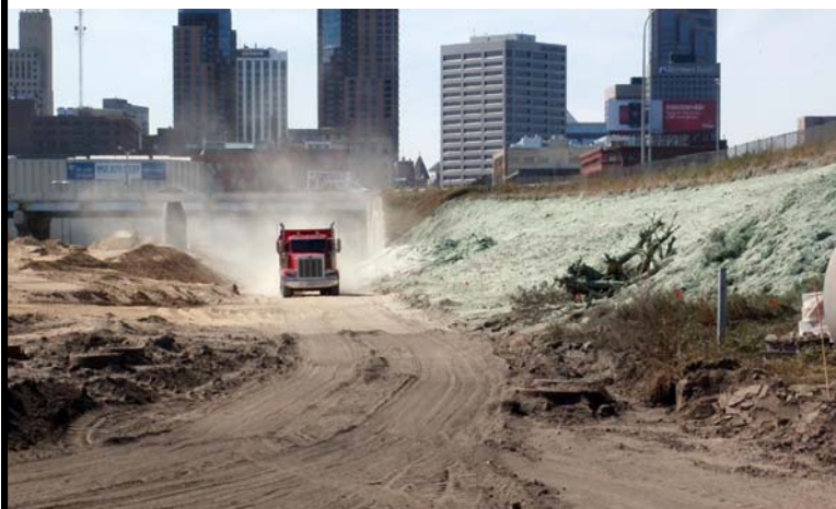
Fugitive dust loss to off-site targets in urban and rural projects. Even though water was applied to photo on right, it was not effective in controlling dust generation
