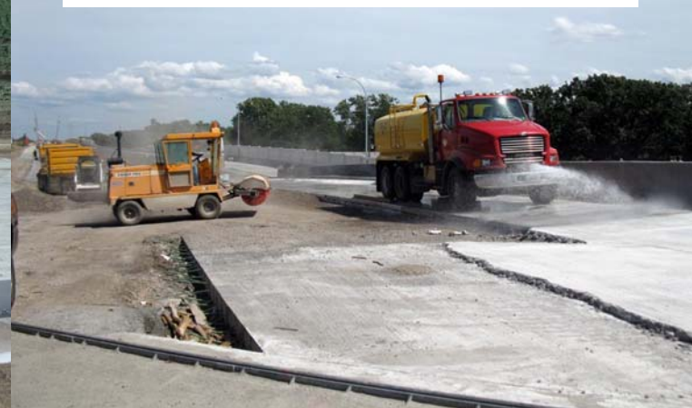
BMP 2. Apply appropriate water from pressure tank to saw fitting (University Ave Light Rail)
