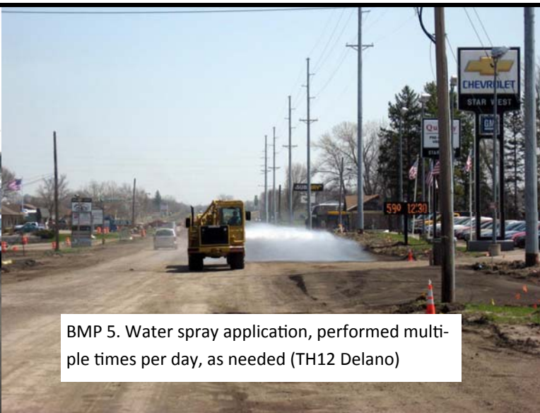
BMP 5. Water spray application, performed multiple times per day, as needed (TH12 Delano)
