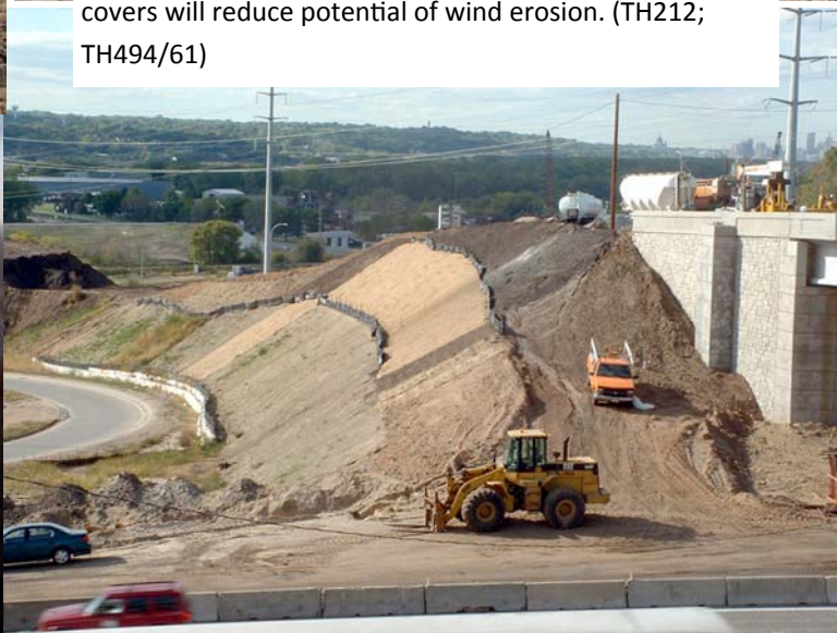
BMP 9. Example installation of a high performance hydraulically applied bonded fiber matrix. Length of service life determines mulch type and applied pounds.
