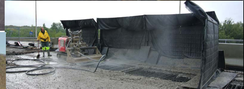
BMP 4/5. Mobile panel wind and mist shroud for pavement demolitions.
