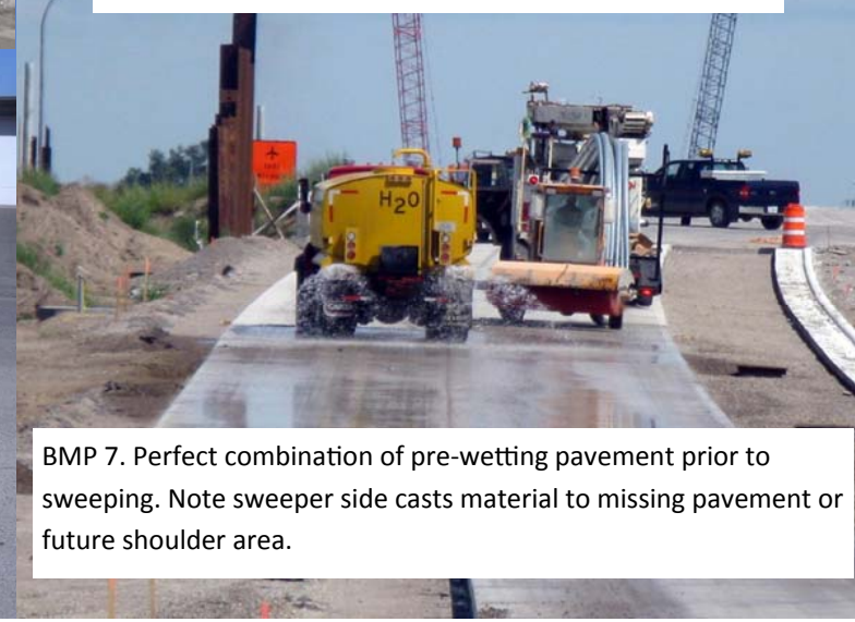
BMP 7. Water spray clean dust generating material from pavement surface. Cementitious materials once dried are difficult to remove by sweeping. (I35W Crosstown)
