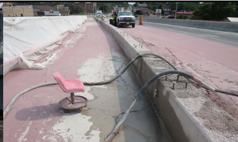
BMP 2. Water blast spray deflected control area using plastic over railing. Note granite blast agent actively swept and water washed clean.
