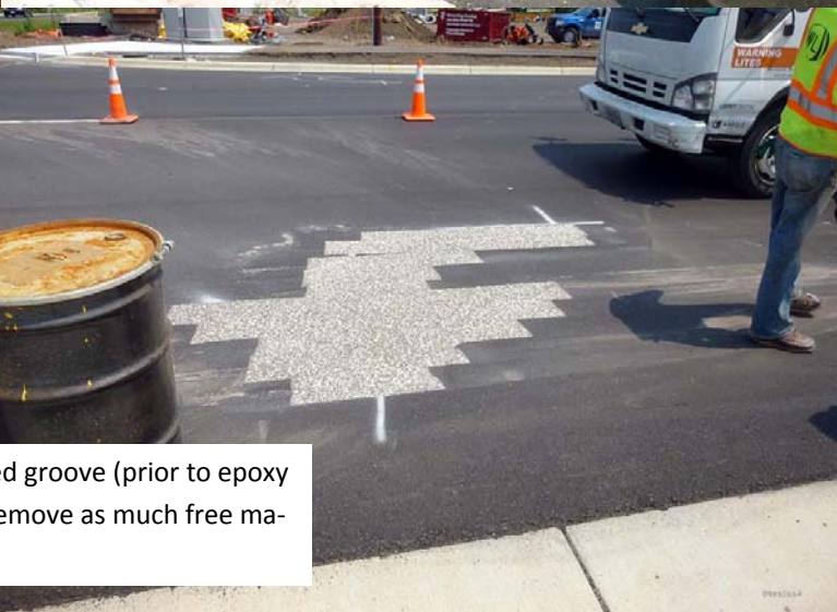
BMP 5. High pressure water jet removal of epoxy or mastic in groove. Complete vacuum removal of all waste and pavement.
