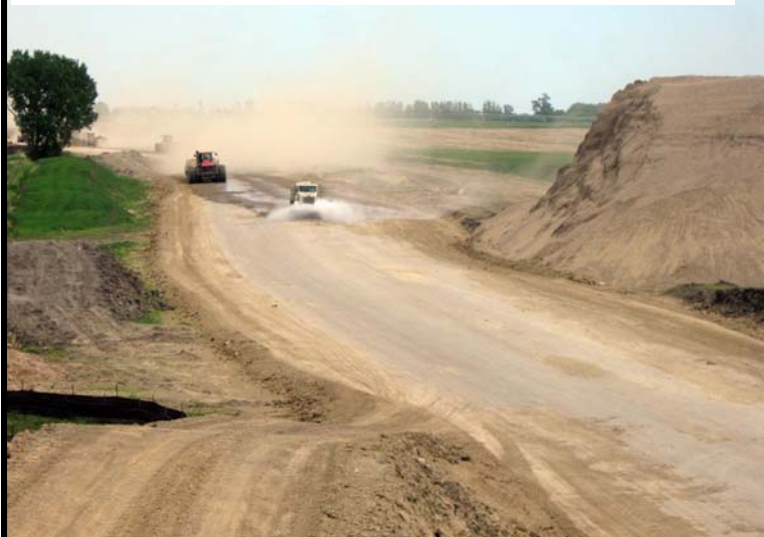
Fugitive dust loss to off-site targets in urban and rural projects. Even though water was applied to photo on right, it was not effective in controlling dust generation
