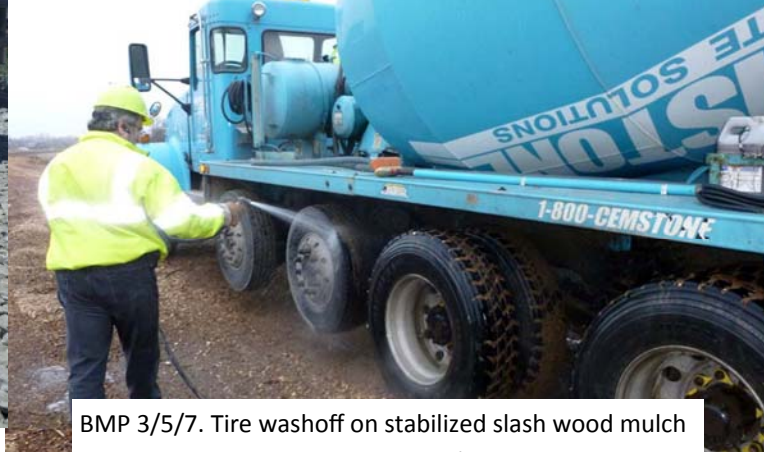
BMP 3/5/7. Tire washoff on stabilized slash wood mulch haul road and exit to TH51 (TH694/Snelling Ave).
