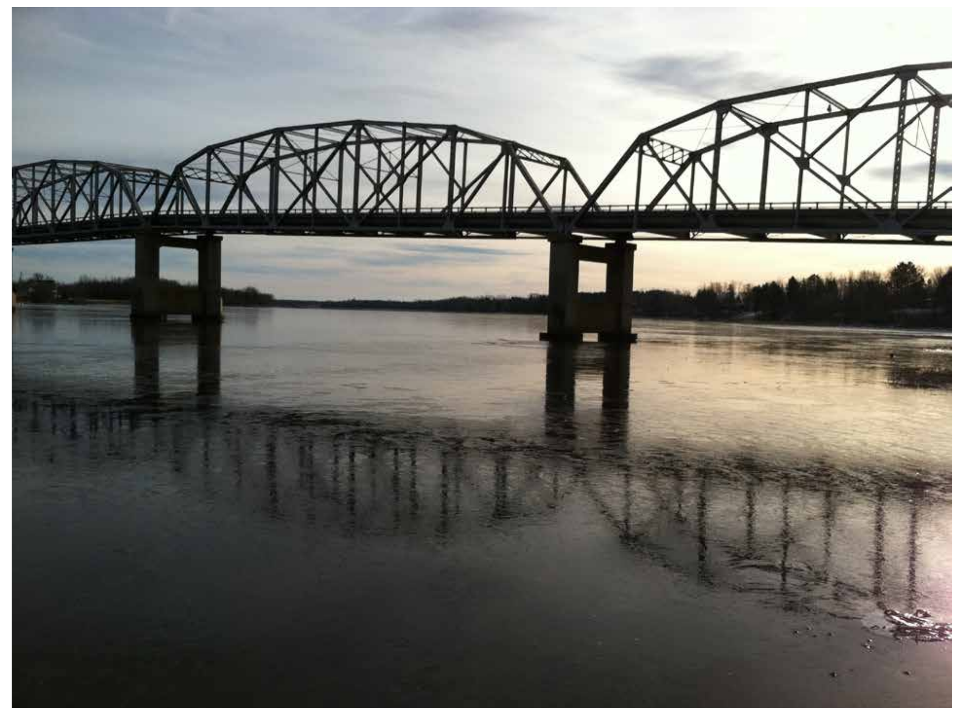
Figure 2: Removal of Historic Bridge will be mitigated as defined in the Memorandum of Agreement
