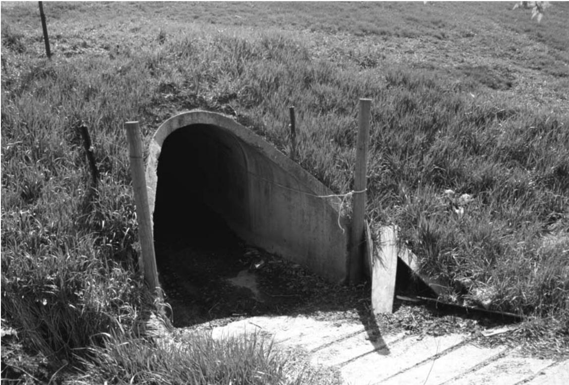
This poured concrete animal underpass in central Minnesota is approached by a scored concrete walkway. The walkway provides traction for animals and reduces erosion on the steep slope. Stearns County, 2004. (Gemini Research photo)
