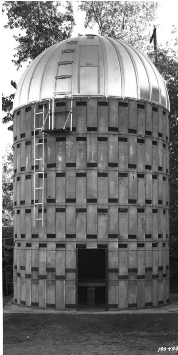
Cement stave corncribs were first built in the 1910s. This brand new example was photographed in 1949. It had steel reinforcing hoops, a hatch in the roof for filling, and a lower door for unloading – all typical of the type. The staves incorporated small metal grates that kept rodents from passing through the air gaps. Location unknown, 1949. (MHS photo by Norton and Peel)
