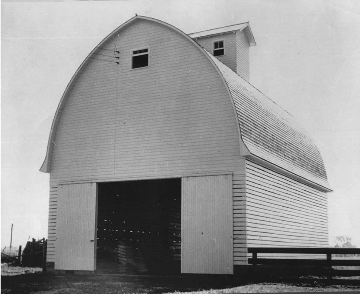
This style of combined corncrib-granary was very popular according to a 1940 publication from *Successful Farming* magazine (Fox 1940). There was a central drive between two cribs on the first level, and overhead grain bins on the second. Judging by the electric wires, there was probably an electric-powered elevator inside. This building was built with glue-laminated arches made by Rilco, a company founded in St. Paul in 1939. Location unknown, 1947. (MHS photo)
