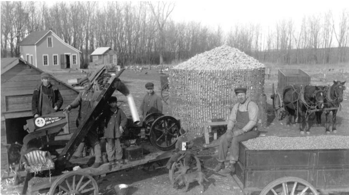
Farmers shelling corn using a sheller mounted on a flatbed. The shelled corn was placed in the wagon (right), and the ear corn into a simple corncrib (background) made of two rows of snow fencing. The two men on the left hold a banner that reads "Let the nation own the trusts," a socialist slogan. Location unknown, circa 1910. (MHS photo by Ole Mattiason Aarseth)
