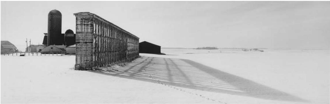
The optimal width for Minnesota corncribs was 6' to 7' but the length could vary. The height was determined first by comfortable hand-filling and then by the height of mechanical conveyors. This long, continuous crib probably had several interior partitions. Corncribs were often aligned north and south to catch cross-winds. Farm near LeCenter, 1998. (MHS photo by Chris Faust)
