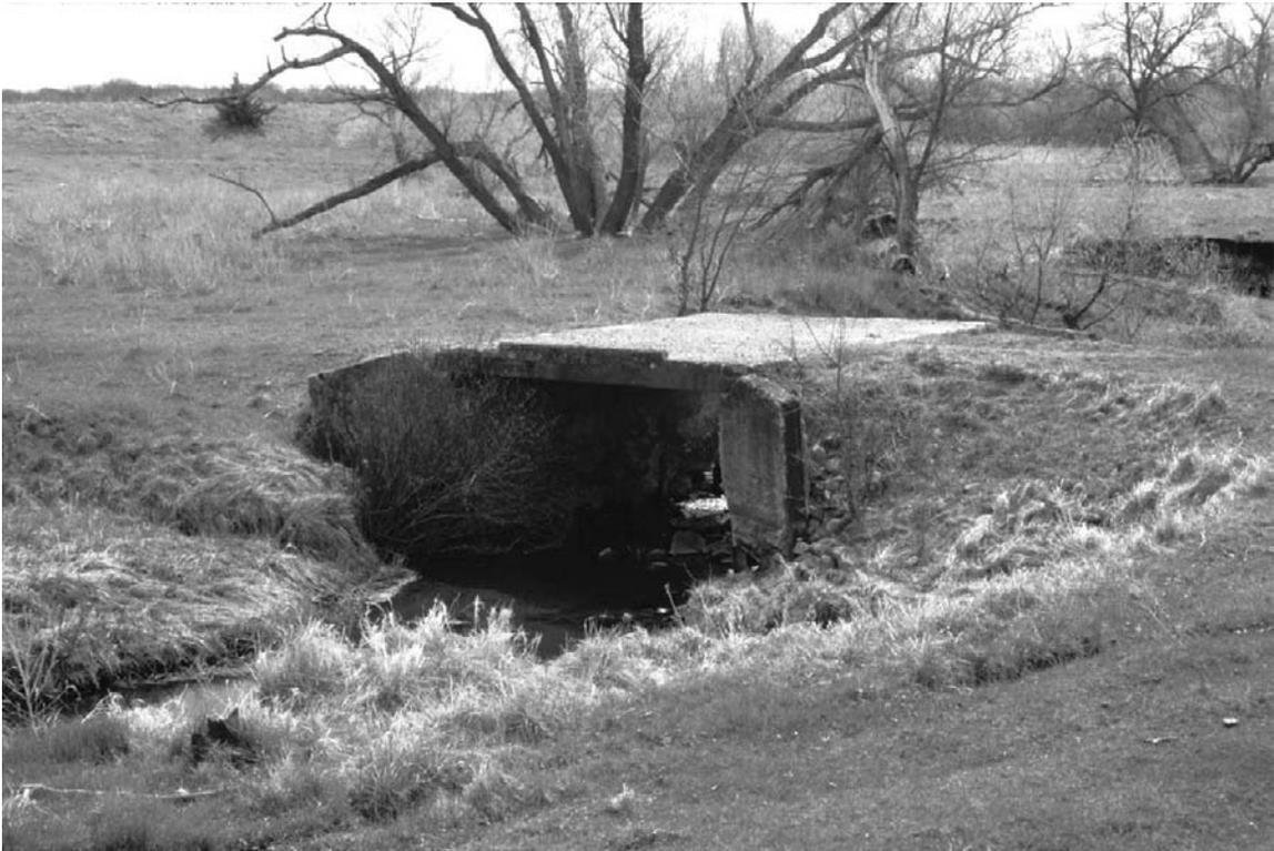
A poured concrete bridge (reinforced with iron) that carries a narrow farm lane over a stream in Stearns County. 2004. (Gemini Research photo)
