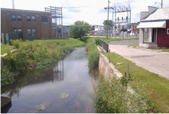
Figure 2: A view upstream from Culvert 5722
