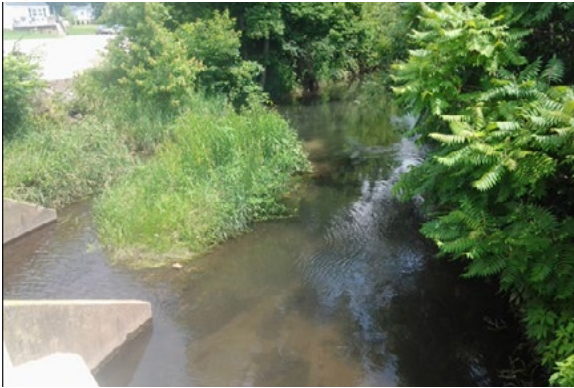
Figure 3: A view downstream from Culvert 5722
