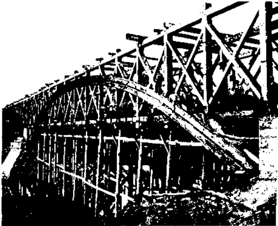
*Figure 1-11.- Burr bridge built in 1848 over the White River at White River Junction, Vermont. This photo was taken as the bridge was being removed in 1890, to be replaced by an iron bridge (photo courtesy of the American Society of Civil Engineers; © 1976. Used by permission).*
