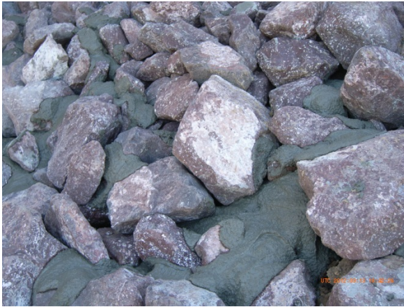
Matrix Riprap close-up during installation, and just after completion
