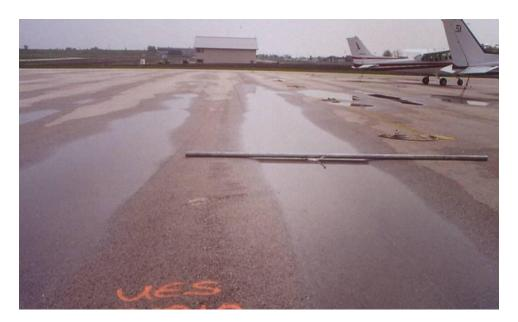
Ruts are localized, load related, areas of pavement having elevations lower than the surrounding sections. Rutting is due to base and subgrade consolidation, caused by excessive wheel loads or poor compaction. Ruts indicate structural failure, and can cause hydroplaning. At low severity, ruts have an
