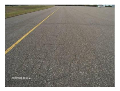
Alligator (or fatigue) cracks are a series of interconnected load-related cracks caused by fatigue of the asphalt surface. Alligator cracking is a significant structural distress and develops only in places subject to traffic loads. These cracks typically initiate at the bottom of the asphalt layer (where tensile strains
