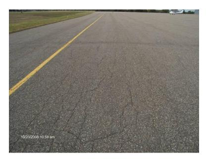
Alligator (or fatigue) cracks are a series of interconnected load-related cracks caused by fatigue of the asphalt surface. Alligator cracking is a significant structural distress and develops only in places subject to traffic loads. These cracks typically initiate at the bottom of the asphalt layer (where tensile strains
