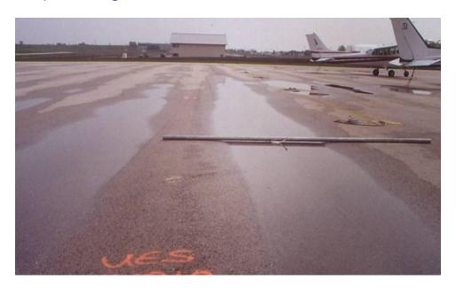
Ruts are localized, load related, areas of pavement having elevations lower than the surrounding sections. Rutting is due to base and subgrade consolidation, caused by excessive wheel loads or poor compaction. Ruts indicate structural failure, and can cause hydroplaning. At low severity, ruts have an
