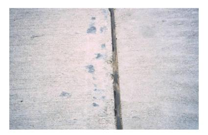
Joint seal damage is recorded at three severities: low, medium, and high. When joint sealant is in perfect condition (no damage), it is not a distress. At low severity, at least 10 percent of the sealant is debonded but still in contact with the joint edges (i.e., joint sealant is in serviceable condition but should
