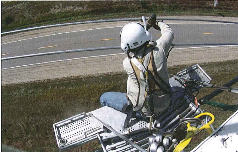
Working from a platform attached to a helicopter, a utility lineman attaches a spacer between transmission conductor.
