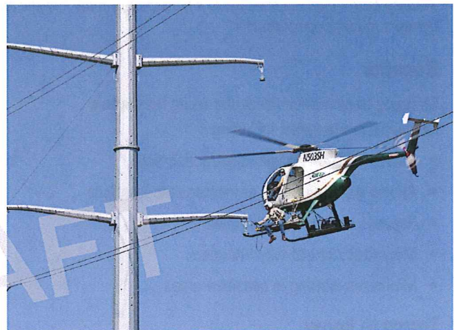
Above. A utility lineman attaches a spacer between transmission conductor.
