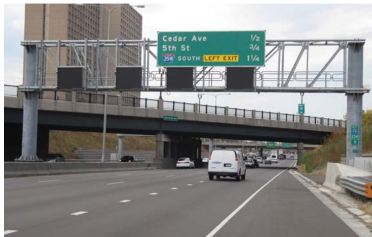
Type OH Sign - Sign Bridge (Design C)
