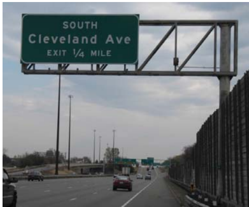
Type OH Sign - Cantilever (Design A)
