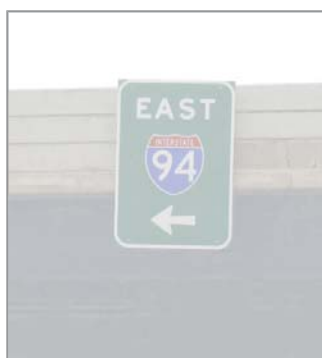
Type D Sign Bridge Mounted
