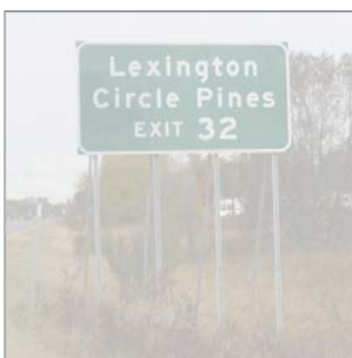
Type D Sign Ground Mounted
