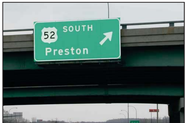
Type OH Sign - Bridge-Mounted
