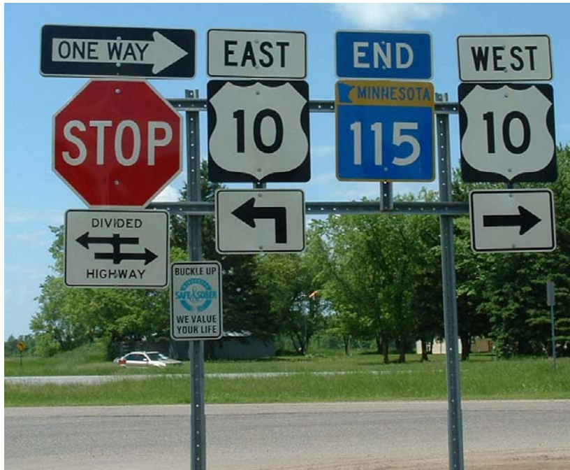
FIGURE 3-4 STOP Sign and Route Marker Assembly
