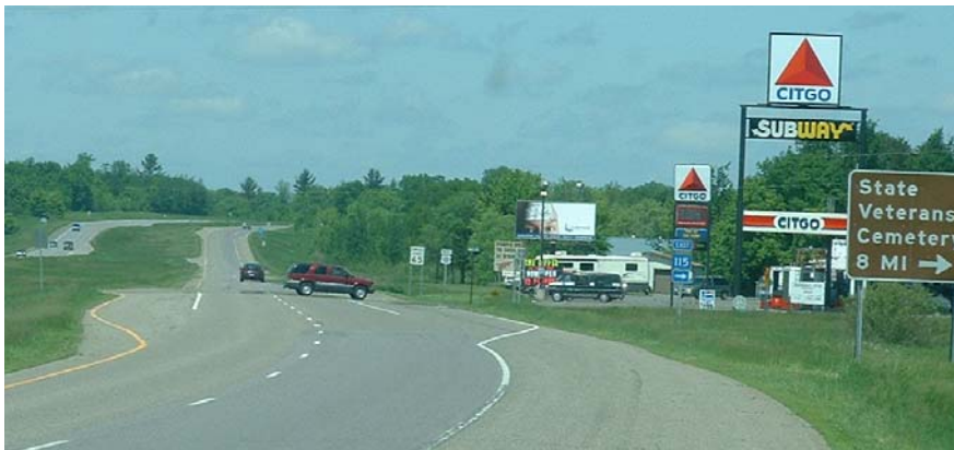
FIGURE 3-2 TH 10 Left and Right Turn Lanes are Unmarked (NB approach to TH 115)
