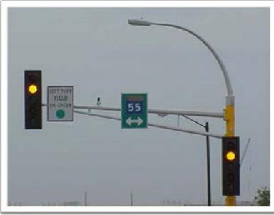
These pictures show a protected/permissive left turn signal. Left turn vehicles are allowed to operate as a protected movement during the green arrow and as a permissive movement (yield to oncoming traffic) during the green ball. Notice the supplemental 'Left Turn Yield on Green' sign.
