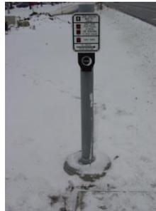
The pedestrian signal face is illustrated with as an arrow. The face is numbered as you approach the intersection with Number 1 being the first on the right and Numbers 2, 3, and 4 as you proceed through the intersection. The labels are preceded by a P with the controller phase number (for example P4-3, P4-4, etc.). The pedestrian push button is labeled with a PB and the controller phase number.
