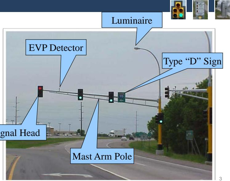
This picture identifies a mast arm pole and some of the common components found on it. This includes emergency vehicle preemption (EVP detector), traffic signal heads (protected and permitted), a luminaire for lighting the roadway and a Type "D" guide sign.
