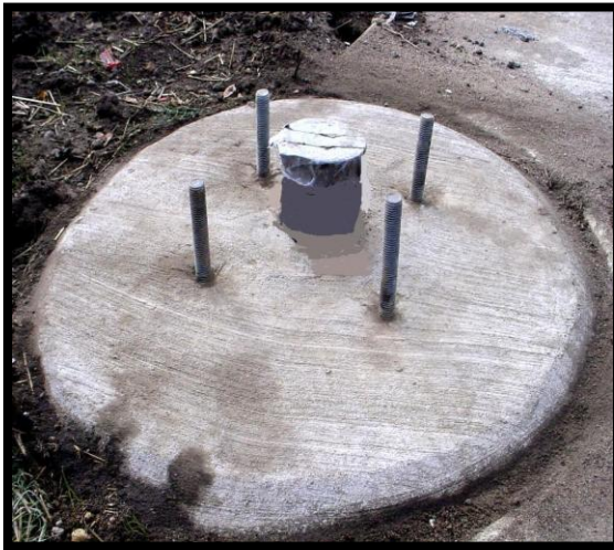
Pedestal Concrete Foundation
