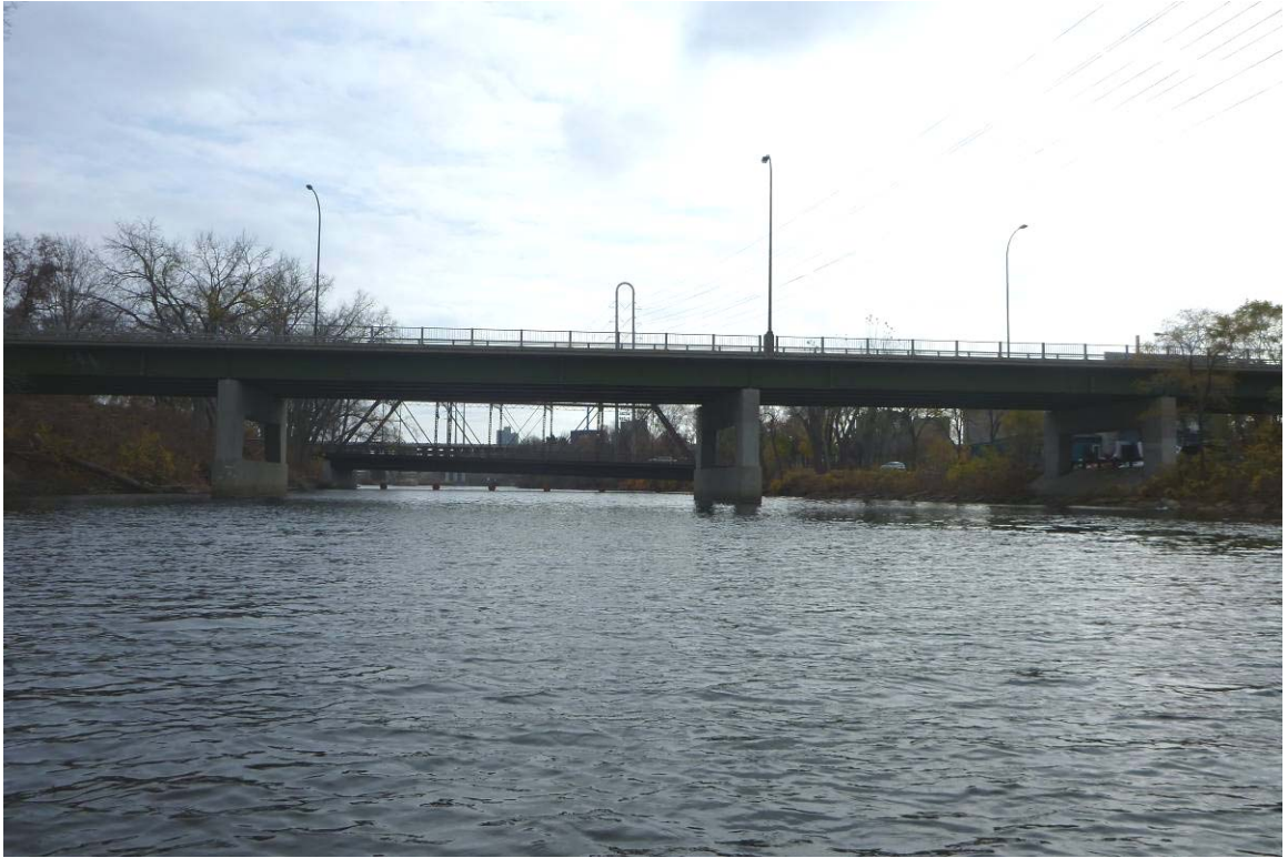
Photograph 1. Overall View of Structure, Looking South.
