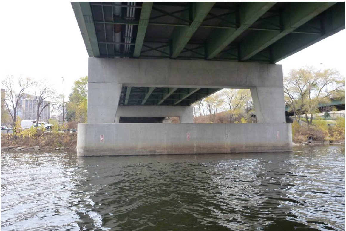
Photograph 2. View of Pier 2, Looking West.
