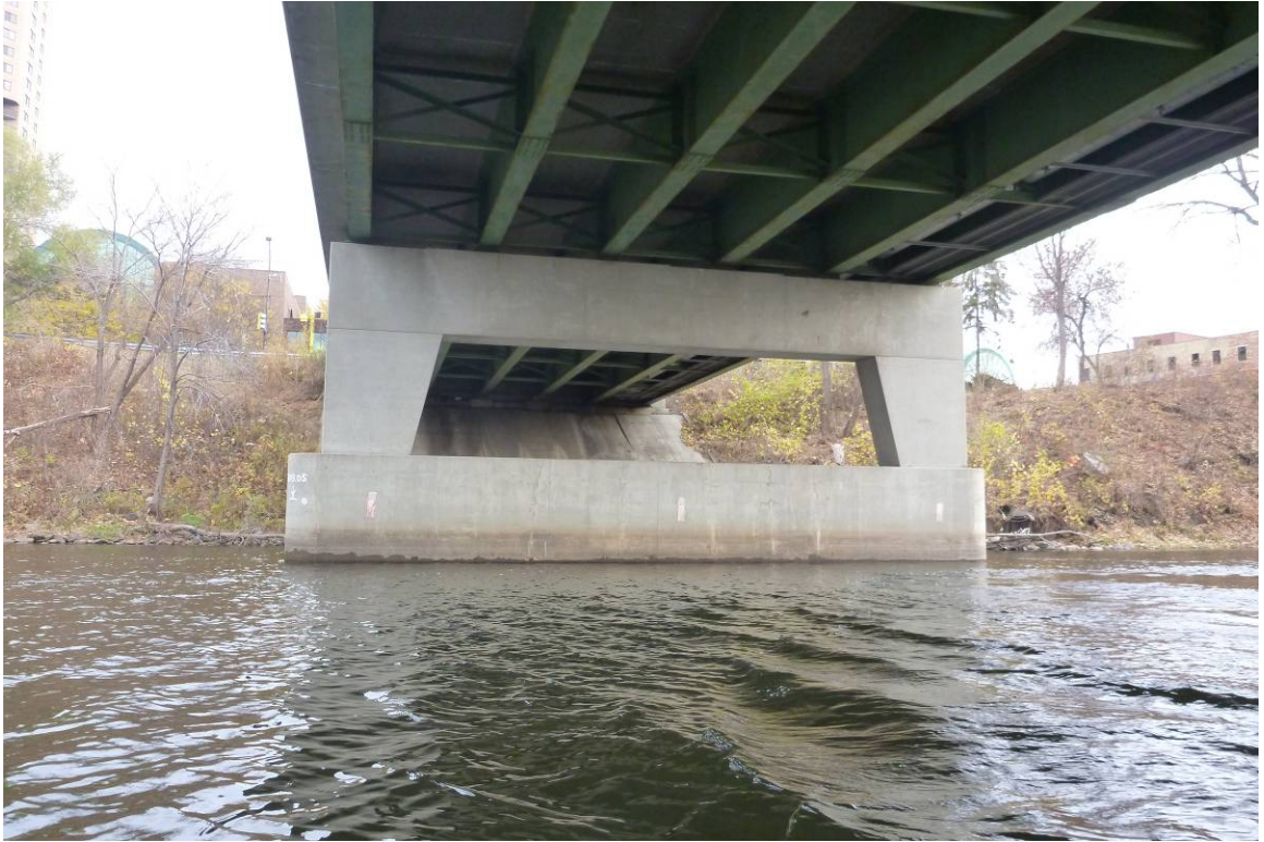
Photograph 3. View of Pier 3, Looking East.
