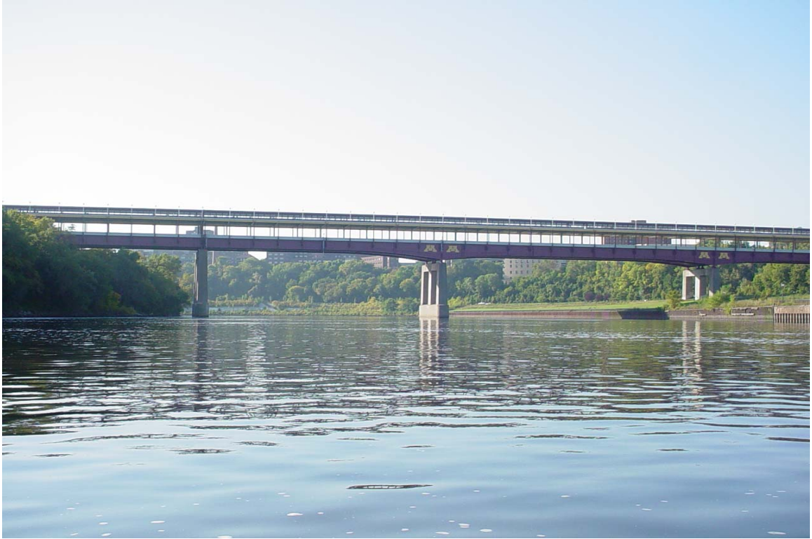
Photograph 1. Overall View of the Structure, Looking South.
