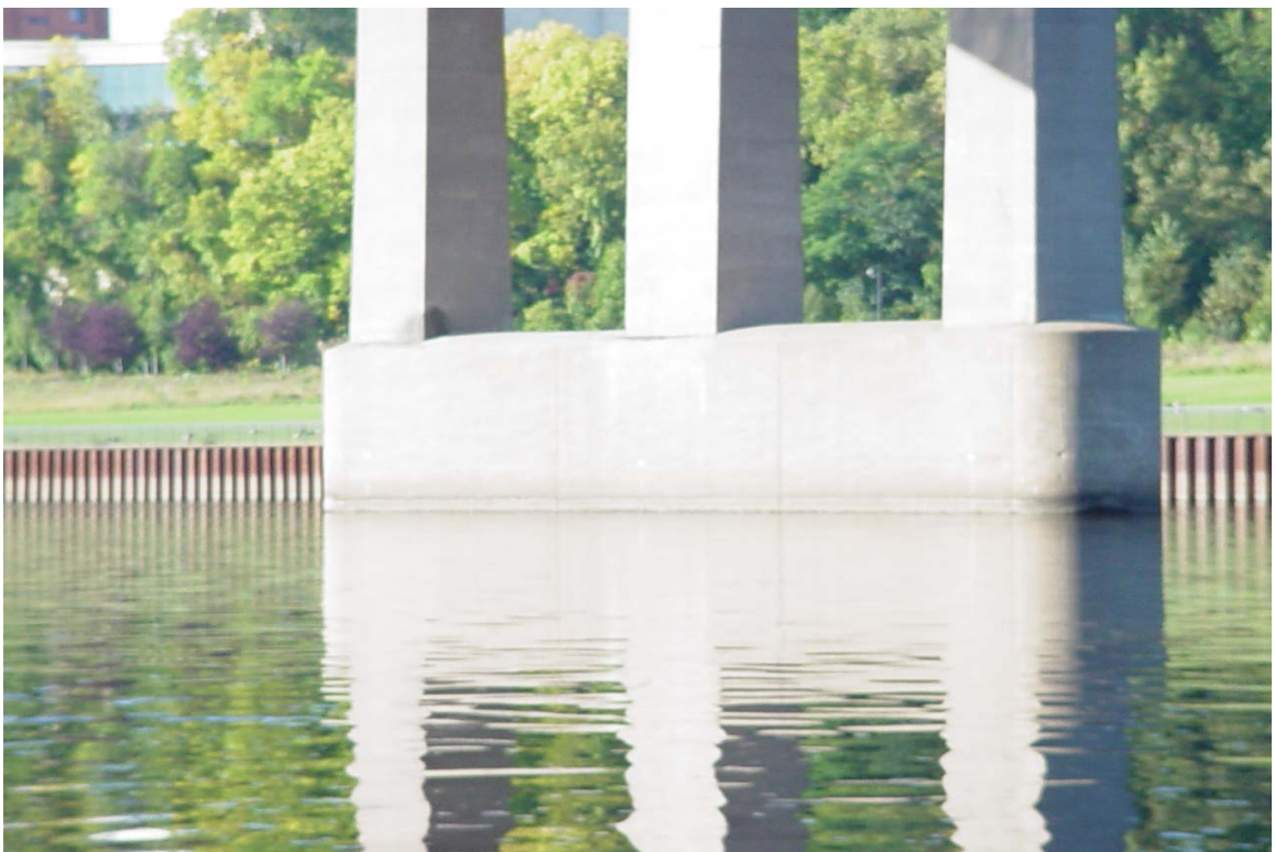
Photograph 2. View of West Pier, Looking Southwest.
