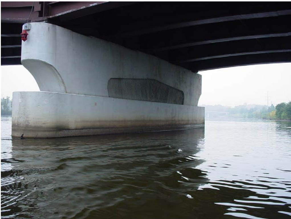
Photograph 2. View of Pier 1, Looking Southeast
