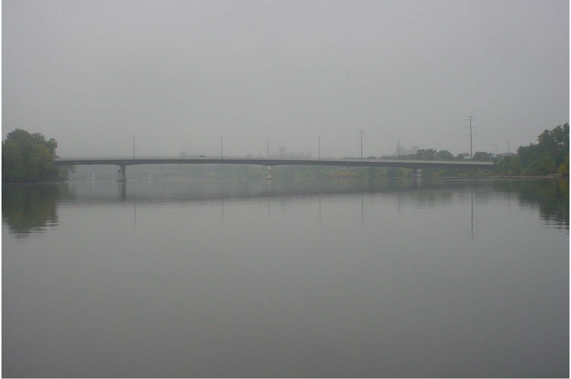
Photograph 1. Overall View of the Structure, Looking South.
