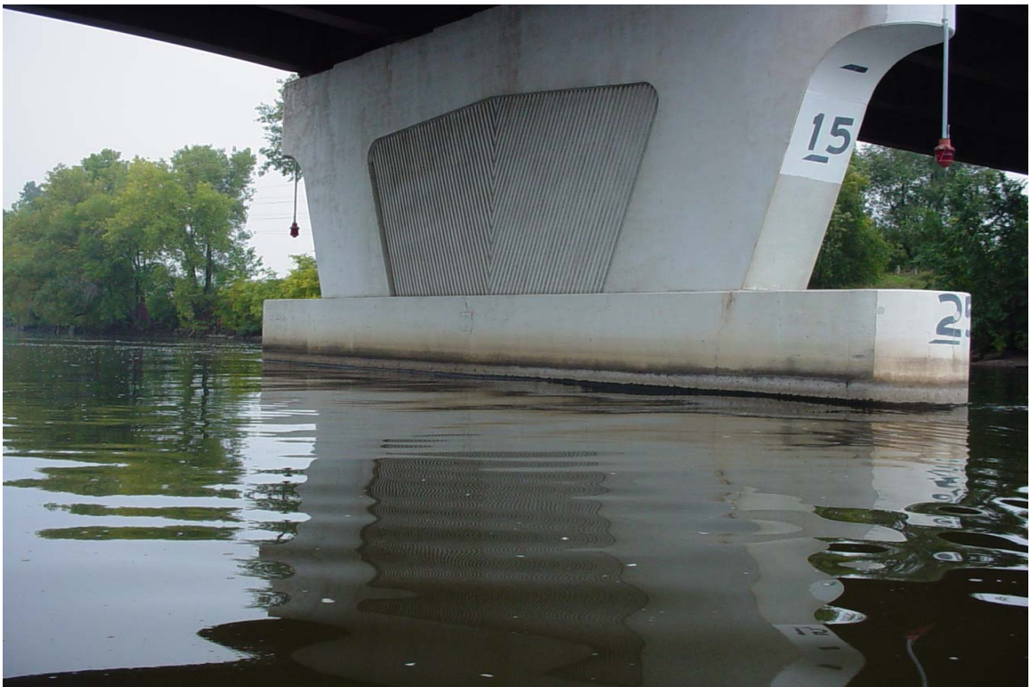
Photograph 4. View of Pier 3, Looking Southwest.
