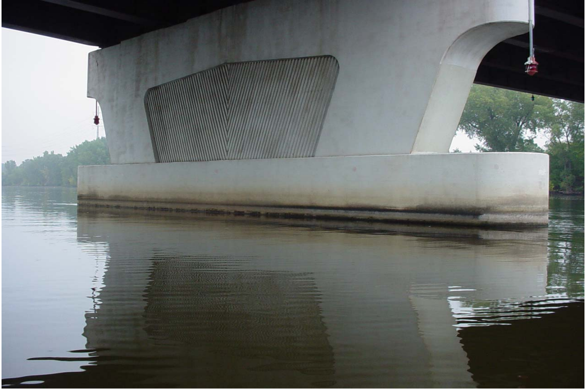
Photograph 3. View of Pier 2, Looking Northeast.
