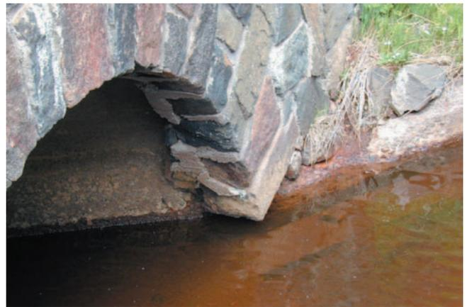
**S** Erosion under south wall arch
