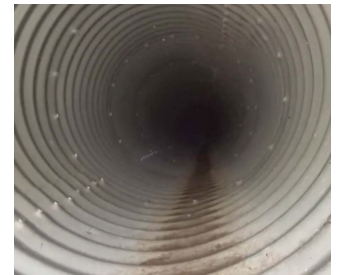
End of pipe inspection
