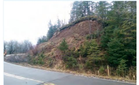
In a significant rainfall, a shallow slope failure like this one along County Highway 210 in Carlton County can lead to extensive cleanup and road detouring.
