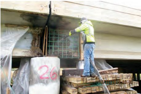
which is sprayed from a hose. Testing repaired and unrepaired girders from the bridge showed that this technique successfully repaired severely deteriorated beam ends for a \$5,000 to \$10,000 investment. MnDOT is continuing to refine this method and will continue to use the beam end repair method if similar conditions are encountered in the state.
