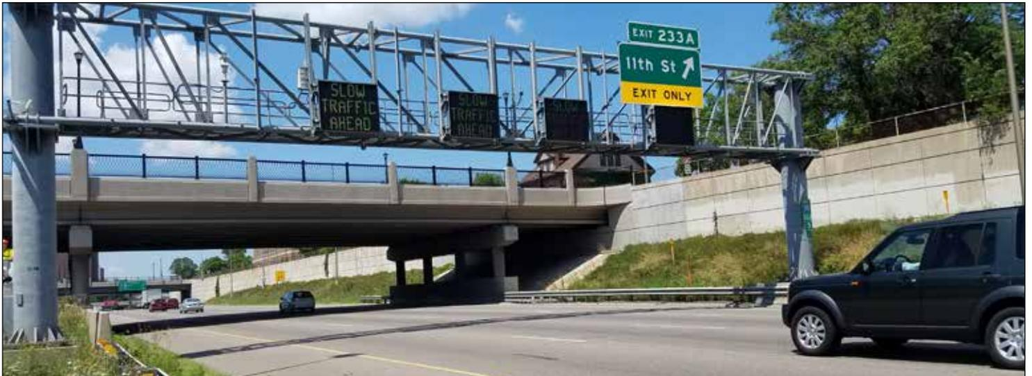
The new queue warning system involved two sets of changeable message boards attached to gantries above I-35W and I-94.
