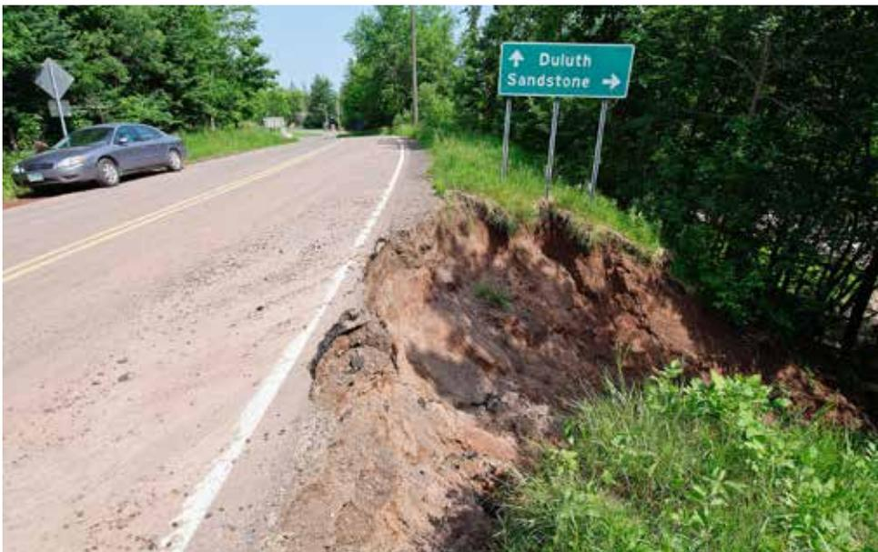
Flash flooding can cause costly damage to state highways. By identifying slopes that are vulnerable to slides, MnDOT can target areas for embankment work as part of future highway projects. (Photo by Dave Gonzalez)
