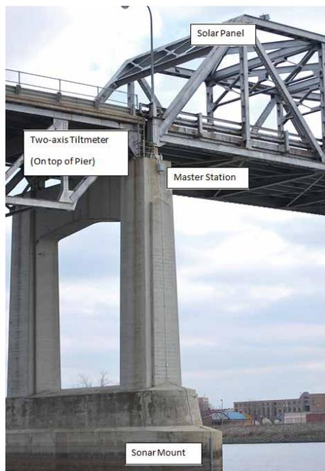
**Bridges & Structures** — A leading cause of bridge failures is bridge scour, where water erodes riverbed soil around abutments or piers. MnDOT already sends inspectors out to monitor bridges judged at risk for failure because of scour, but having a system in place that would continuously monitor such bridges and alert personnel wirelessly when scour reaches a dangerous level would be much more effective, particularly on bridges that are difficult to access during a flash flood.
