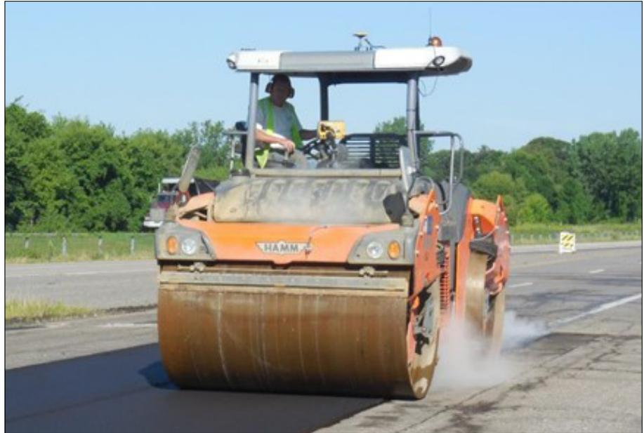
Full compaction was thought to be achieved only under traffic loadings. But a Superpave 5 asphalt mix will be compacted to the design level air voids with regular paving equipment during construction.
