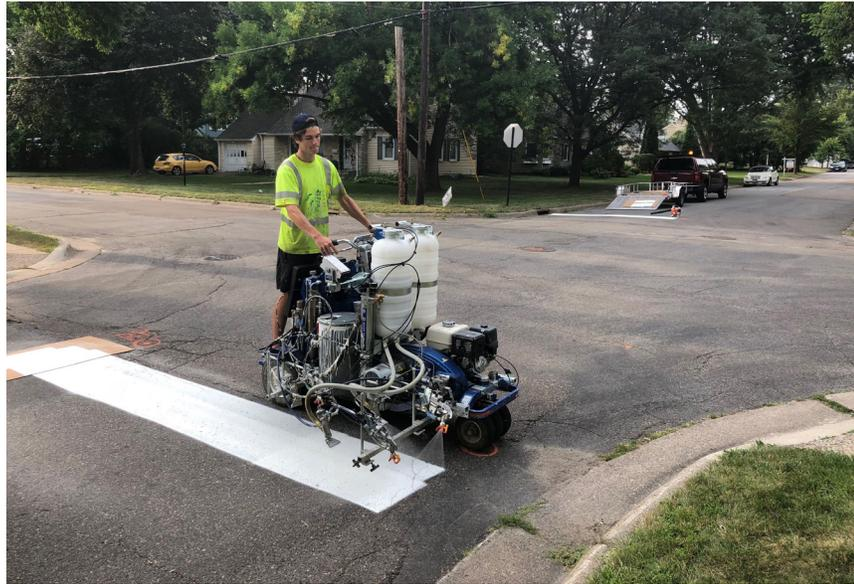
Researchers installed stop lines at 23 intersections as part of an observational before-after field study. Video of drivers’ responses to the new stop lines were compared to previous recordings of the intersections without the stop lines.
