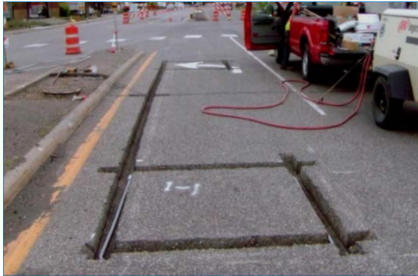
Loop detectors are installed in the pavement and incorporated into the system through complex electrical connections. Traffic flow data is collected every 30 seconds and sent to the RTMC.
