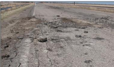
A severely distressed asphalt road in a rural area shows cracking, crumbling, holes and debris.
