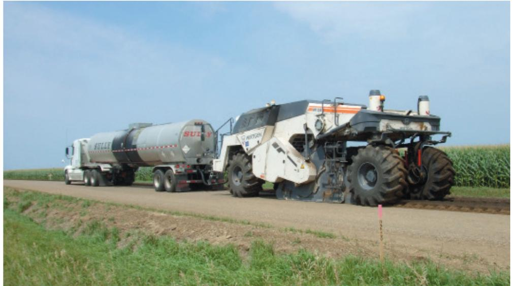
A train of equipment runs on an SFDR site: a tanker of new asphaltic material connected to a reclaimer that pulverizes the old pavement and mixes in part of the road base and possibly stabilizing agents.
