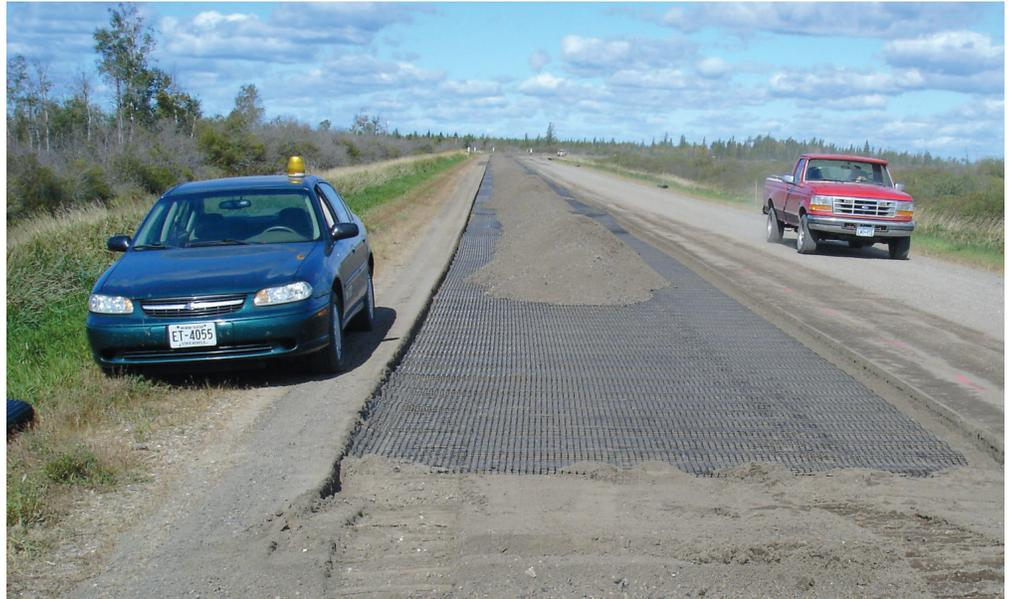
Geogrid is placed between layers of aggregate to stabilize the aggregate layers and improve pavement strength.
