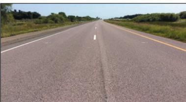
Before and after images of a MnROAD asphalt pavement test section. The stabilized full-depth reclamation section (bottom) shows no cracking after 10 years of service at double the expected design load.
