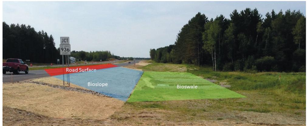
Bioslopes and bioswales provide a natural mechanism for meeting national and state pollution regulations, which require retaining the first inch of runoff during rainstorms.
