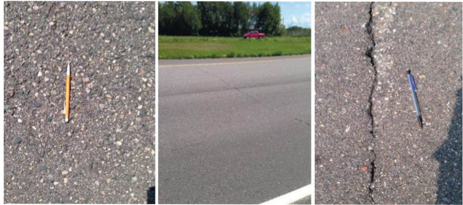
Cracking was extensive for most of the low asphalt binder mixtures. These coarse-graded asphalts prove susceptible to thermal and transverse cracking, and even to potholing from freeze-thaw damage.
